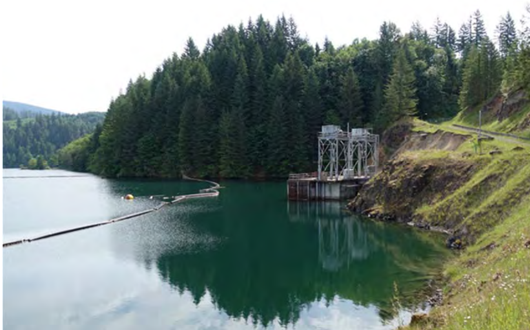
Figure 11. Yale hydro intake structure at high pool.
