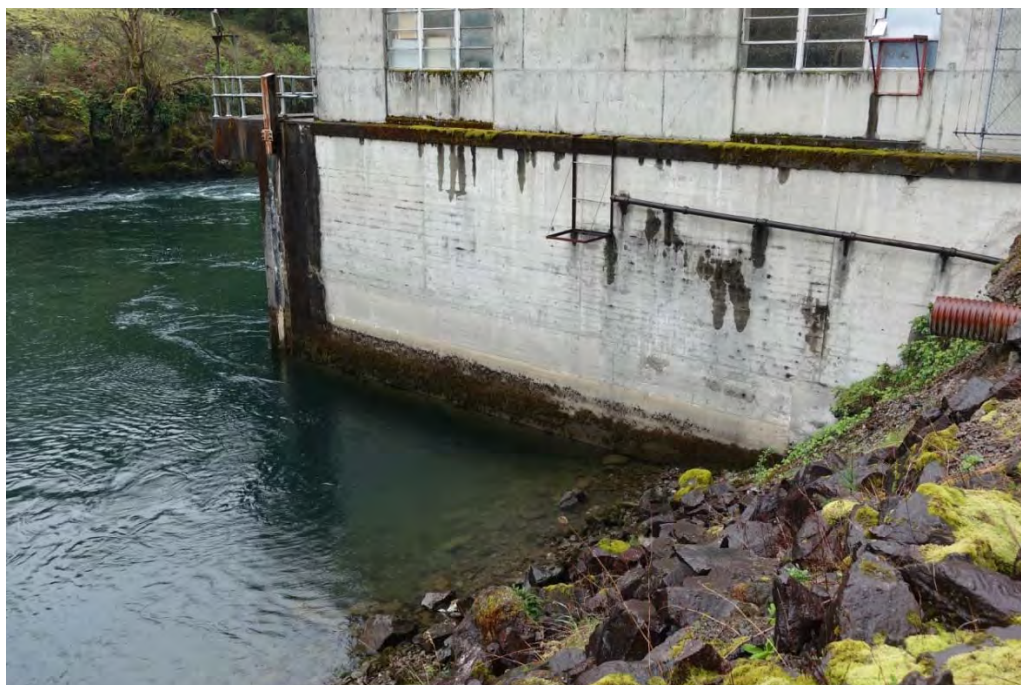
Figure 4. Downstream wall of Yale Powerhouse.
