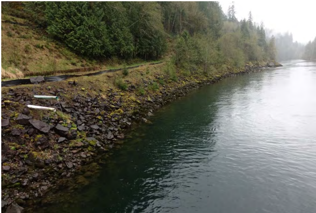
Figure 3. Yale Powerhouse looking downstream.
