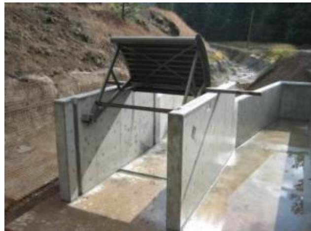
Clearwater 2 Canal Shut-off and Drainage System – Gate Site 2
