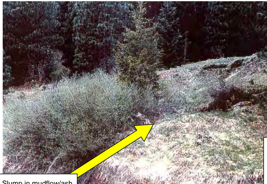
Slump in mudflow/ash deposit on slope above canal
