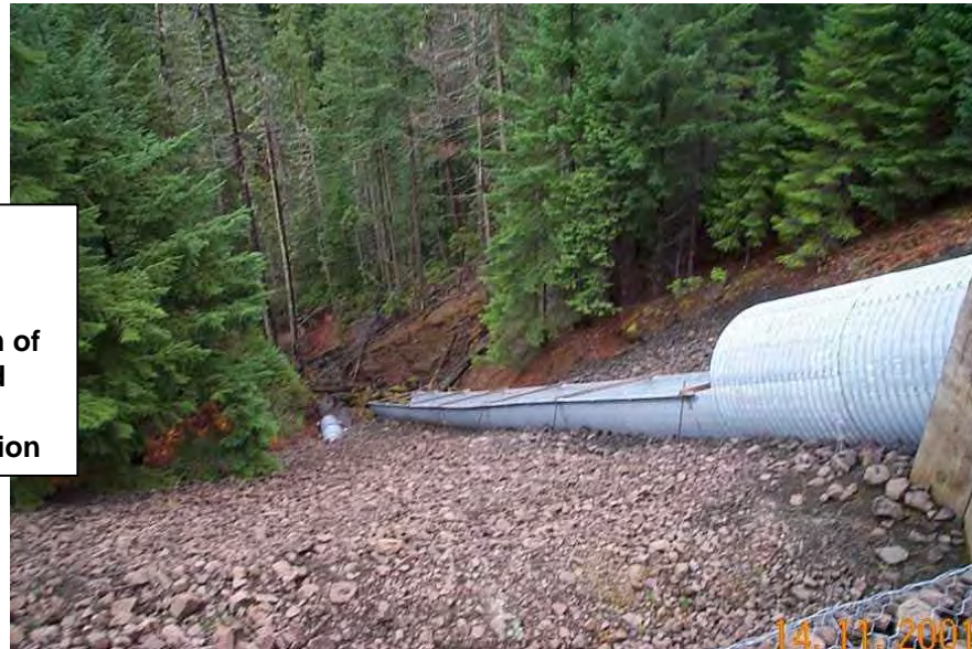
View of Sag Pipe Spillway.
