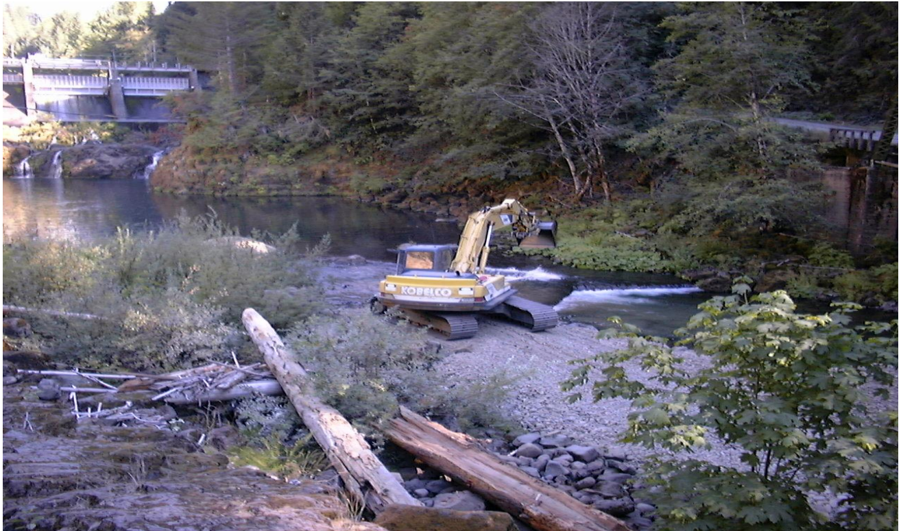
Figure 10. Upper pool during gravel addition in August 2003 (30 cfs) showing the uppermost weir. Note temporary road built of spawning gravel to provide equipment access.
