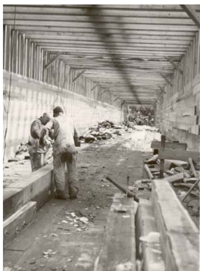
Construction of a diversion flume at Clearwater Dam Site. Toketee, Circa 1949.
