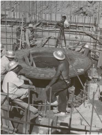
Cement work around a powerhouse draft tube. Circa 1953.
