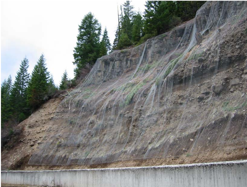
FIGURE 3.2.3-11 Rock Wall Fencing
