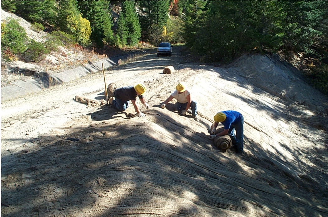
FIGURE 3.2.3-4 Erosion Control Fish Creek
