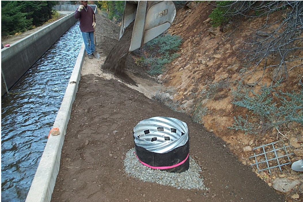
FIGURE 3.2.3-3 Erosion Control Canal Wall Padding Fish Creek
