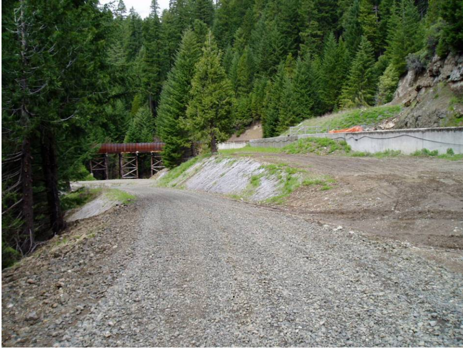
FIGURE D-19 Burma Road — Slide Remediation Near Patricia Creek
