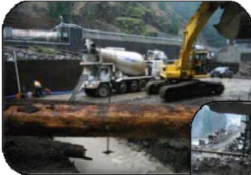
The rebuild involved installing two large, new log weirs in the tailout of the upper pool to hold spawning gravel.
