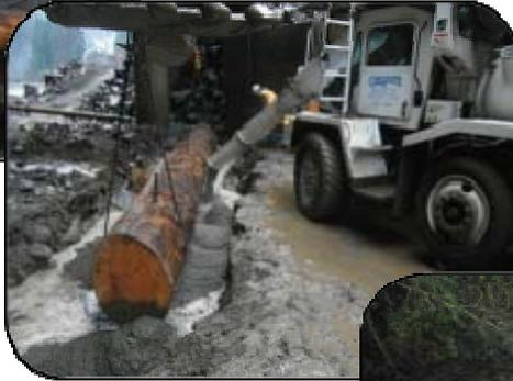
Because these weirs also control the water level of the fish ladder entrance pool, they were surveyed for precision, and thoroughly bedded in concrete for durability. ODFW participated in the design and siting of the weirs. This reconstruction was funded by the fish passage project so did not use any of the dedicated RCC fish habitat funding.
