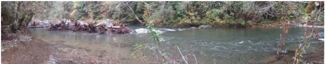
*Site #2 – Root wad/boulder-angled structure slows, raises, and deflects portions of flow into side channel.*
