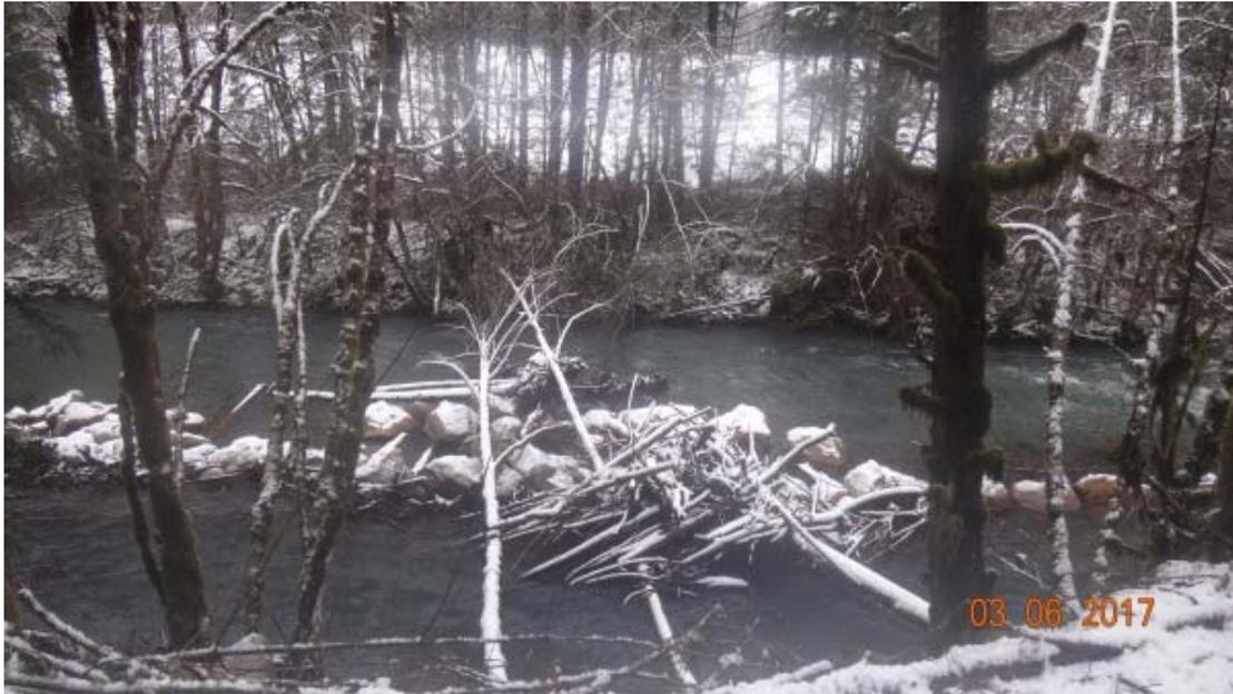
*Site #9 – Root wad/boulder structure oriented perpendicular to both mainstem and reconnected side Channel to slow water and gather woody debris to mimic log jam.*
