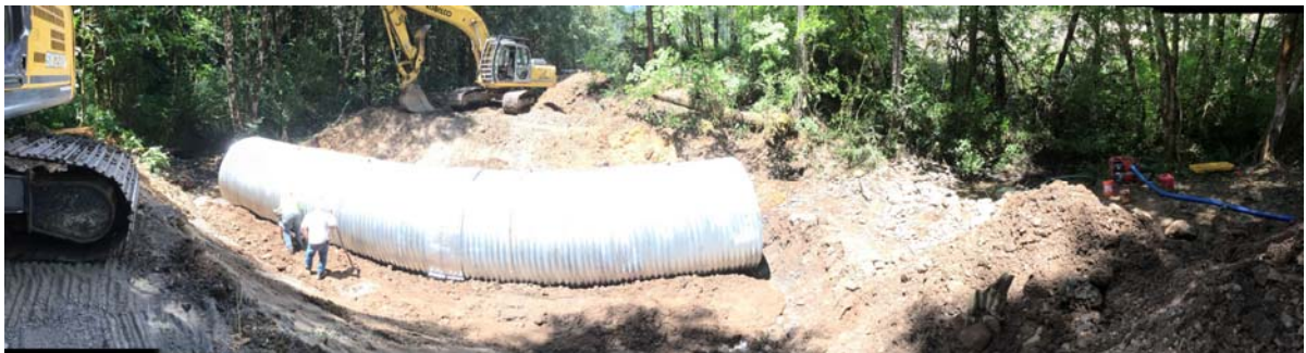
Figure 10. Li'l Conley Creek fish passage culvert upgrade work in progress.
