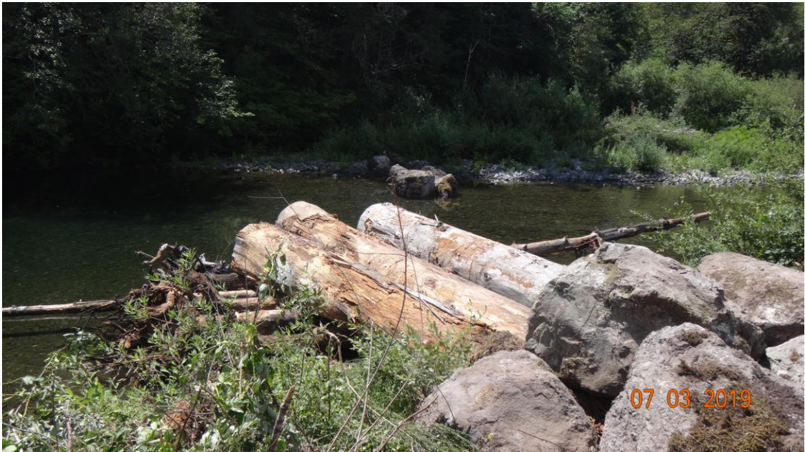
Figure 6. Ballasted log jams provide rearing refuge areas for juvenile salmonids (View 1).
