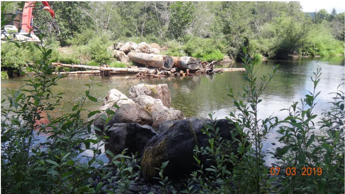
Figure 7. Ballasted log jams provide rearing refuge areas for juvenile salmonids (View 2).
