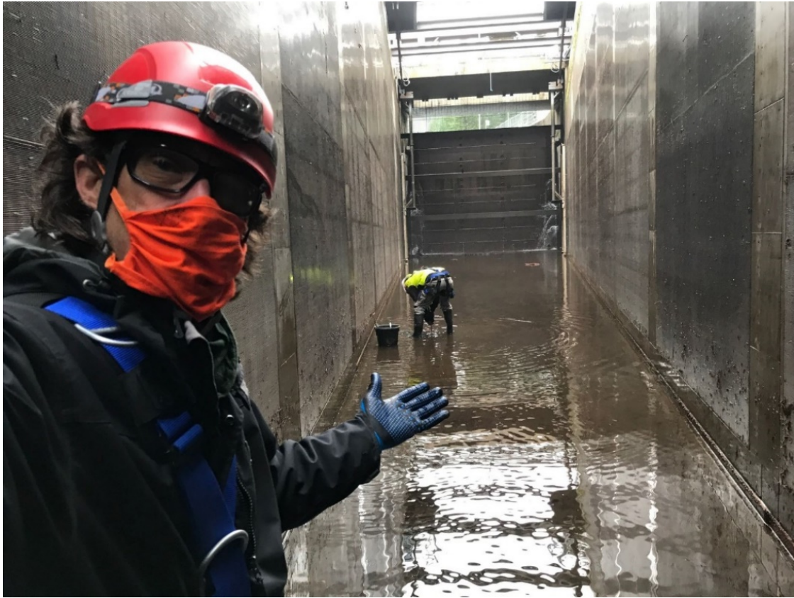
Figure 12. Dewatering the Soda Springs fish screen for planned maintenance.
