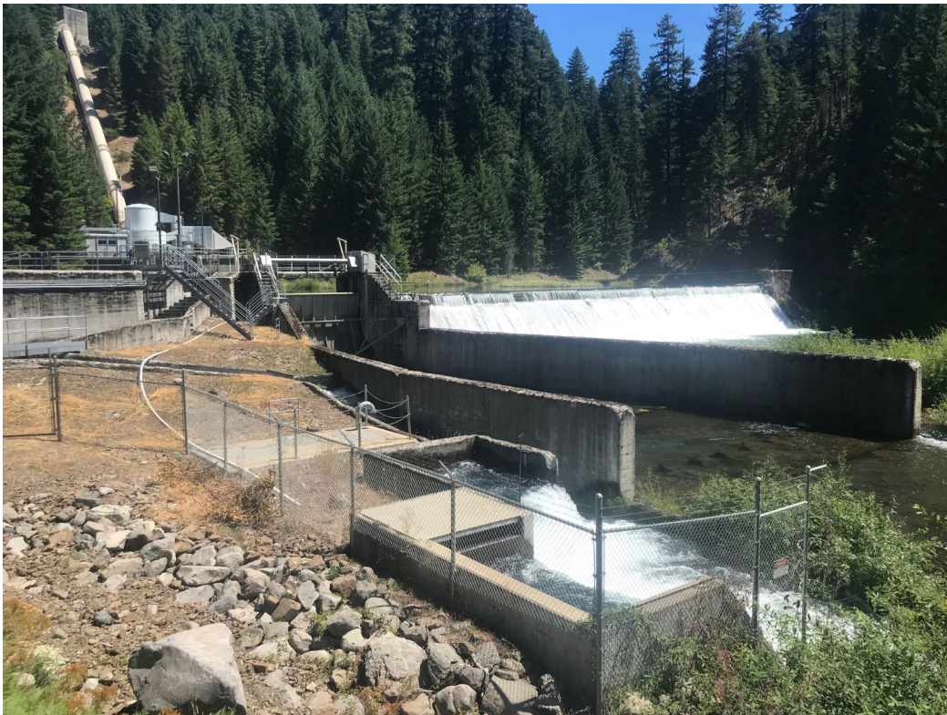
Figure 15. Lemolo 2 Diversion Dam in spill during a planned canal maintenance outage.
