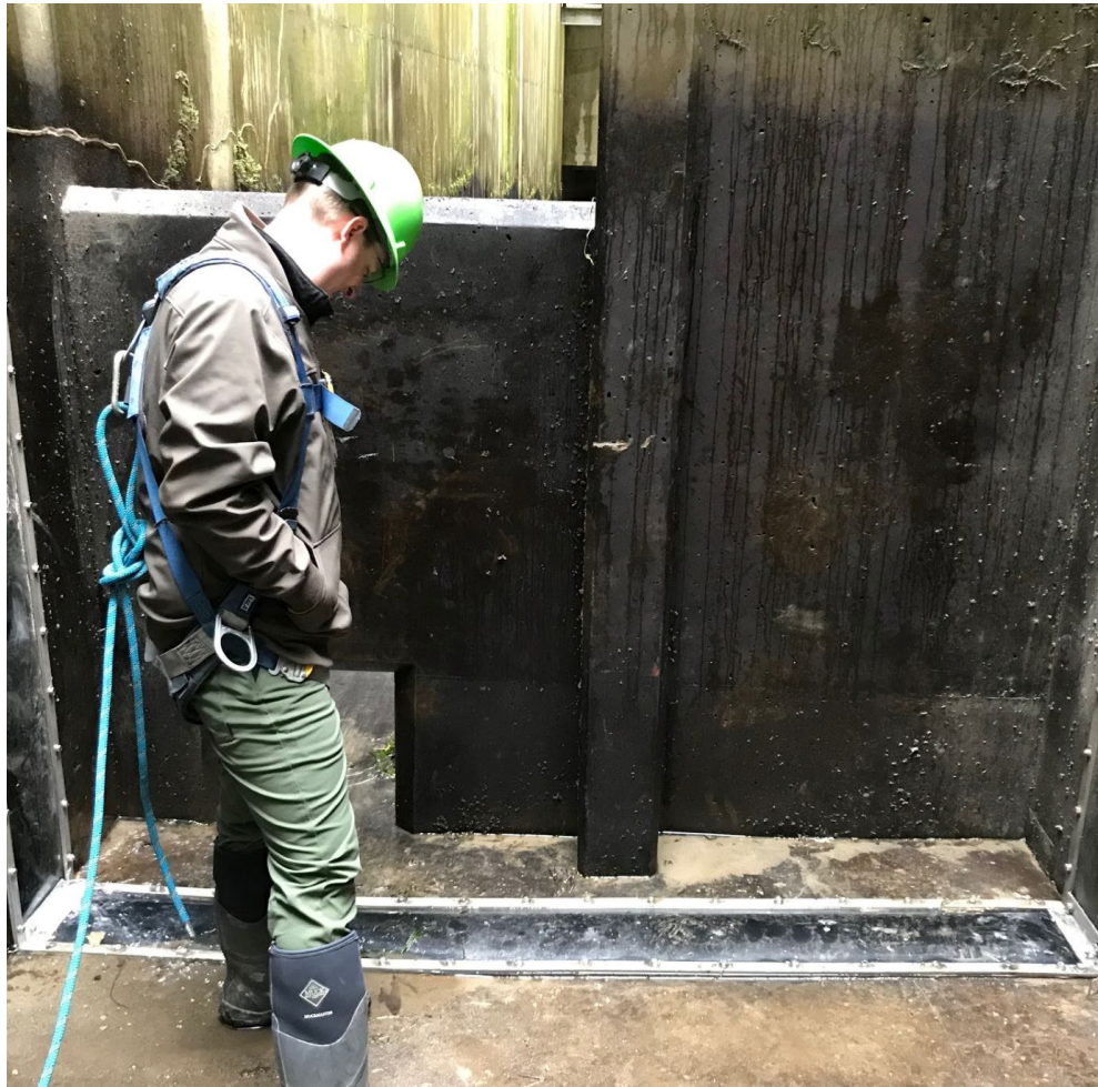
Figure 13. Jason Brandt (ODFW) inspects a new seal along the expansion joint in the Soda Springs fish ladder.
