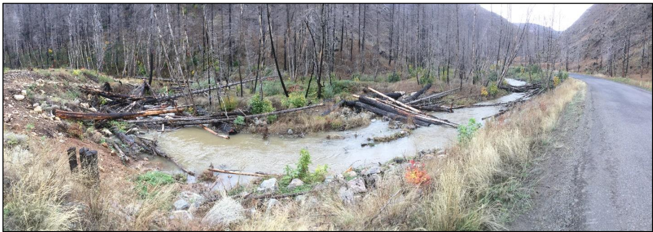
Figure 9. Mechanically-placed, full trees and logs adding 4 log jams within primary, secondary and tertiary channels of East Fork Rock Creek.
