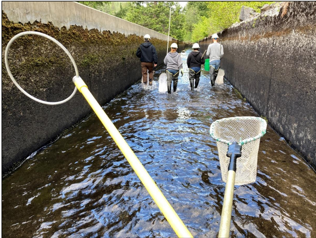
Figure 14. PacifiCorp crew salvaging fish from the Lemolo No. 2 canal during dewatering for planned maintenance, June 2022. The net and electroshocking wand in the foreground are being held by Aquatic Scientist (and photographer) Rich Grost, who is bringing up the rear to shock any fish that get past the primary netters out in front.
