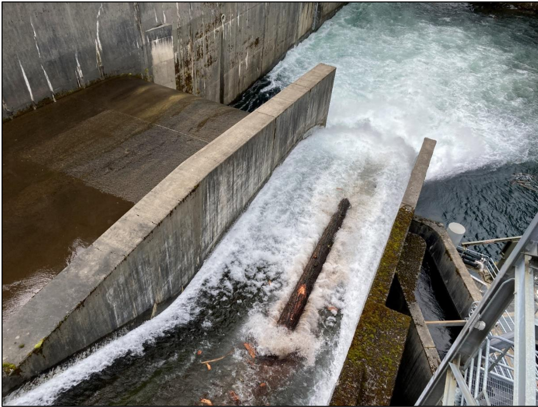
Figure 15. A log being sluiced through the log chute at Soda Springs Dam as part of the Large Woody Debris Passage Program, February 2022.
