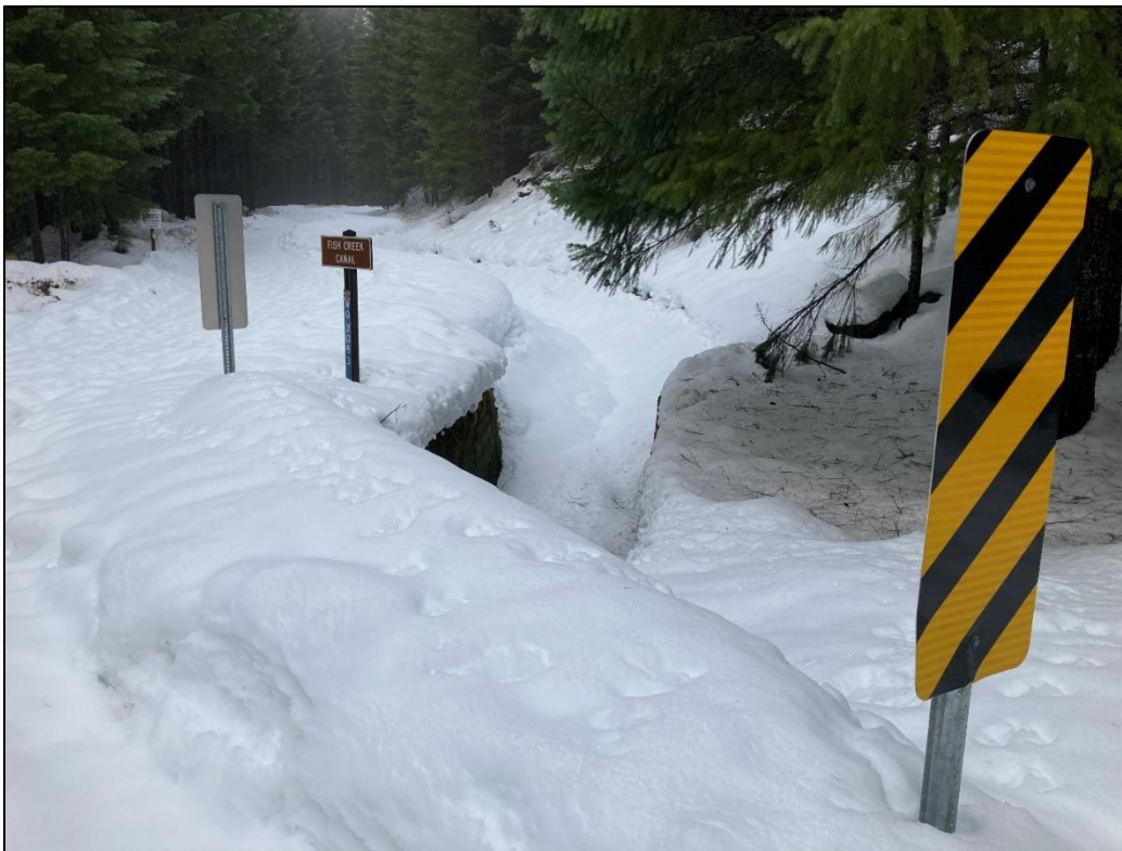
Figure 2. Fish Creek canal buried in snow, January 2022. Due to the high minimum flows required in the bypass reach, diversion of water is often limited to periods of sustained rain and snowmelt.
