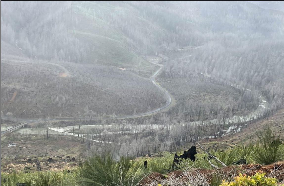
Figure 12. Boulder structures on left dissipating high flow energy while also diverting some water into a large side-channel and the floodplain providing juvenile refugia habitat (flow from left to right of frame).
