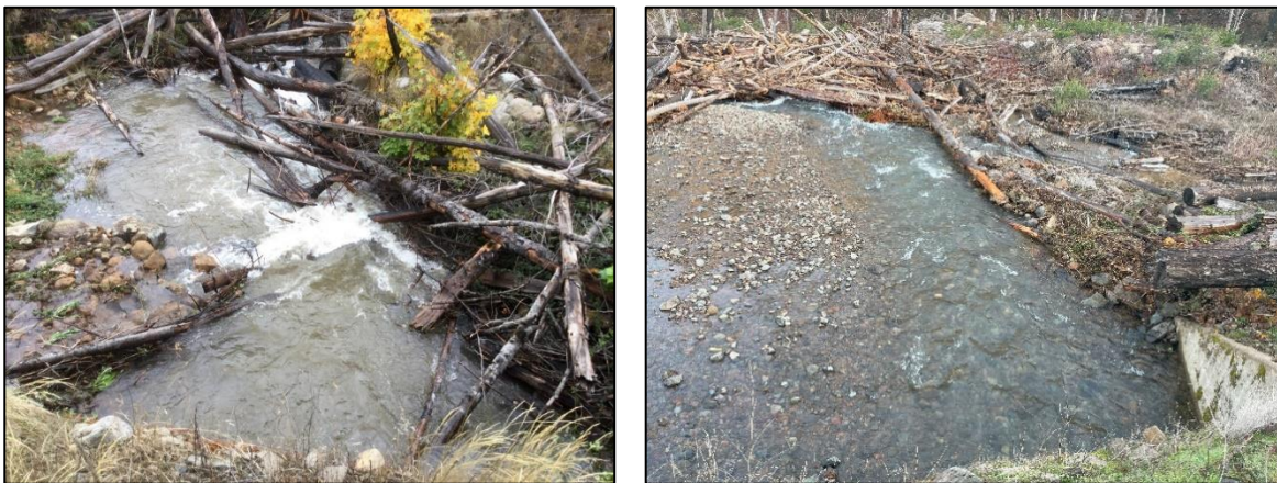
Figure 10. Mace Creek box culvert before (left) and after (right) treatment, illustrating the fish passage improvements.
