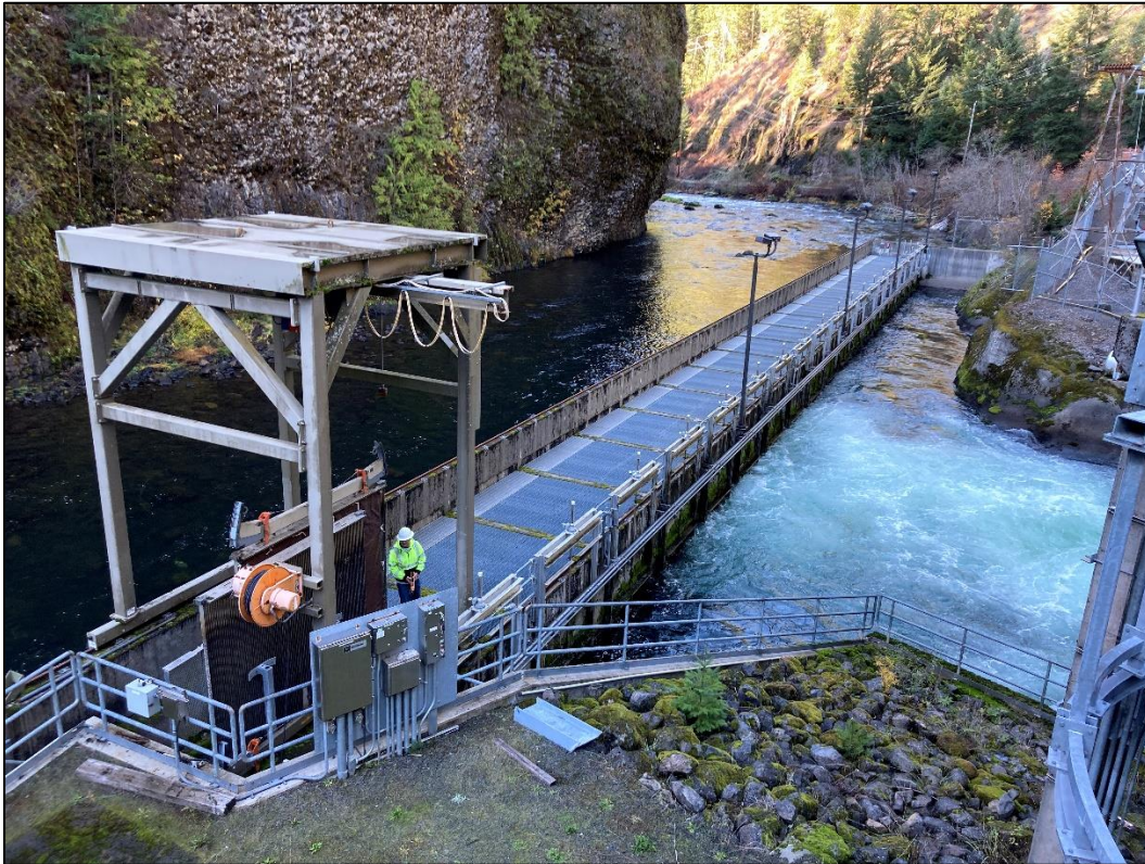
Figure 3. Soda Springs tailrace barrier diffusing the flow and precluding adult salmon and steelhead from the turbulent tailrace (note operator in safety-yellow jacket standing near hoist), December 2023.
