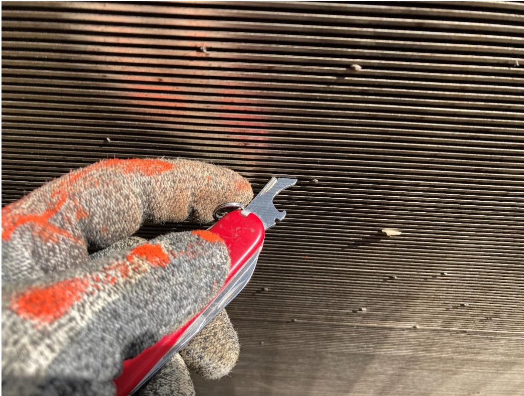
Figure 26. Even a Swiss Army Knife screwdriver is barely thin enough to enter the gaps of the Soda Springs fish screen and dislodge the tiny gravel trapped therein (August 2023).
