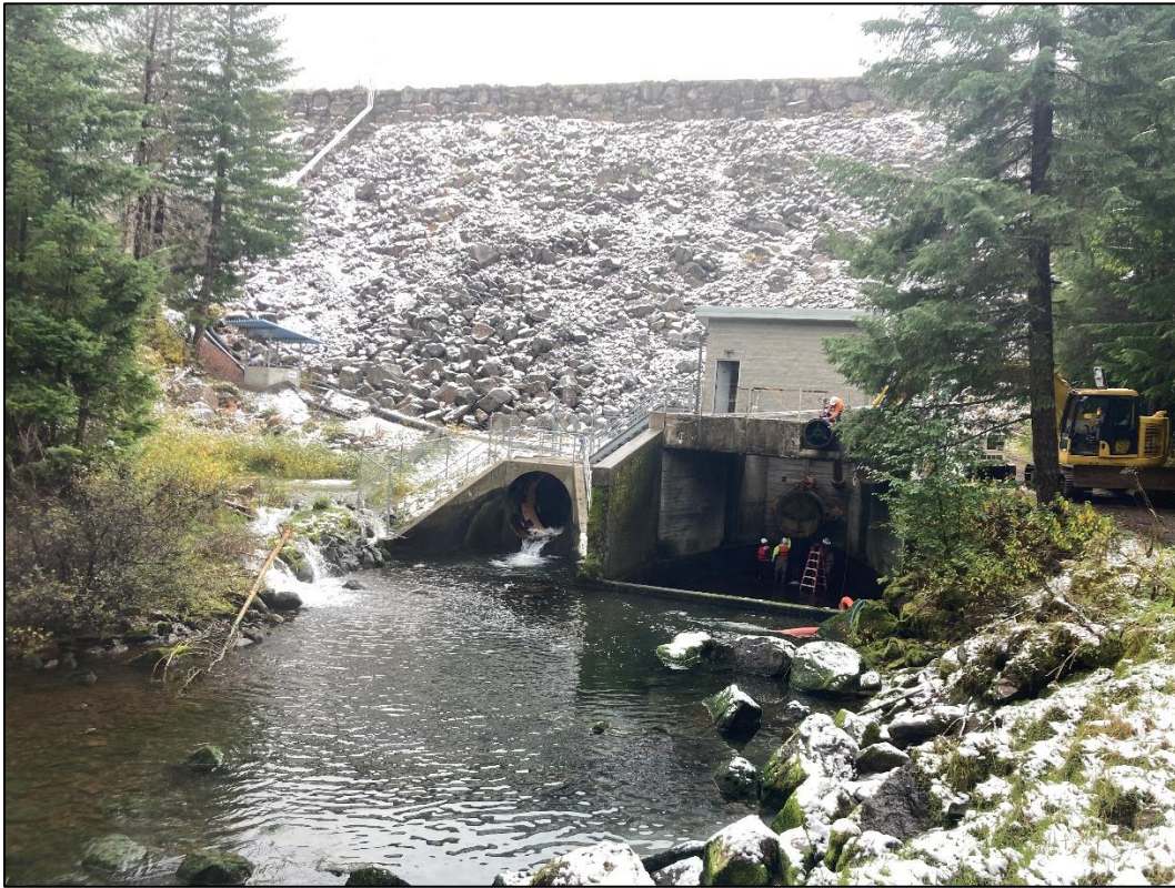
Figure 25. Crews perform a FERC-required inspection of the low-level spill valve at Lemolo 1 Dam, which required RCC approval to modify instream flow requirements downstream of the dam for several days (October 2023).
