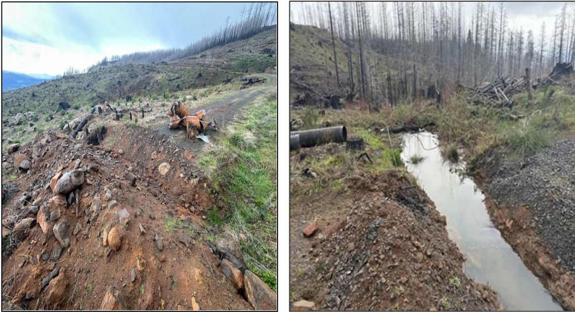
Figure 9. McComas Creek culvert and road decommissioning for erosion and sediment control.
