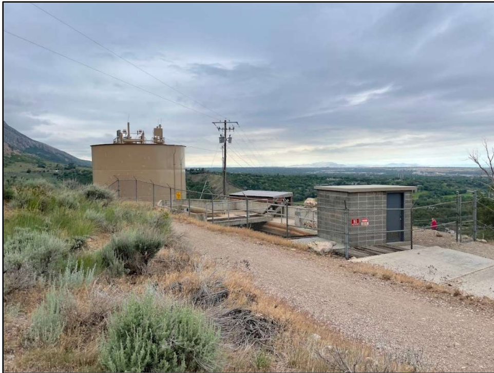
FIGURE 3-3 SHARED-USE SURGE TANK AND NON-PROJECT OGDEN-BRIGHAM CANAL INTAKE
