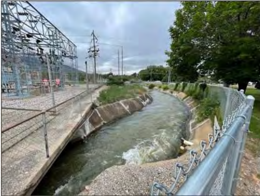
Project Tailrace Canal
