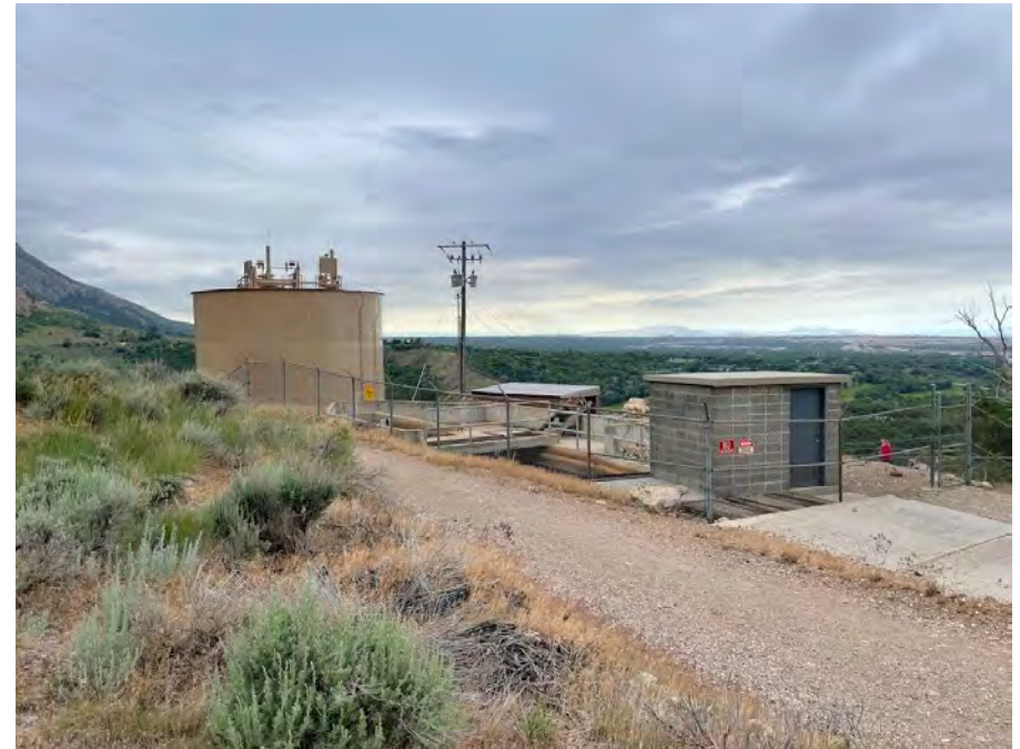
Pioneer Surge Tank
