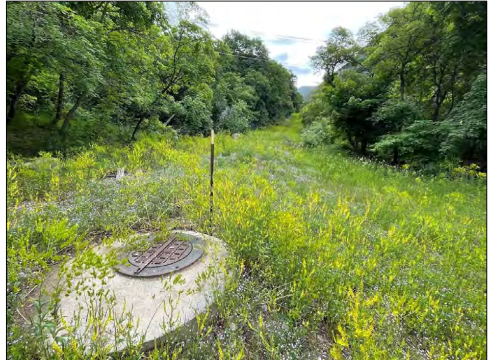
Ogden Canyon Conduit (Buried)
