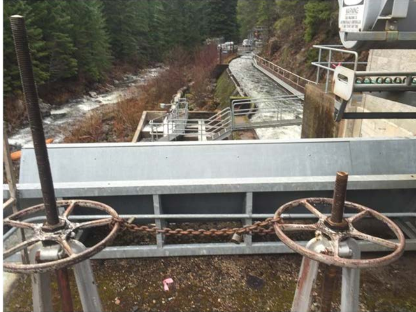
Photo 5. Fish ladder exit orifice gate control
