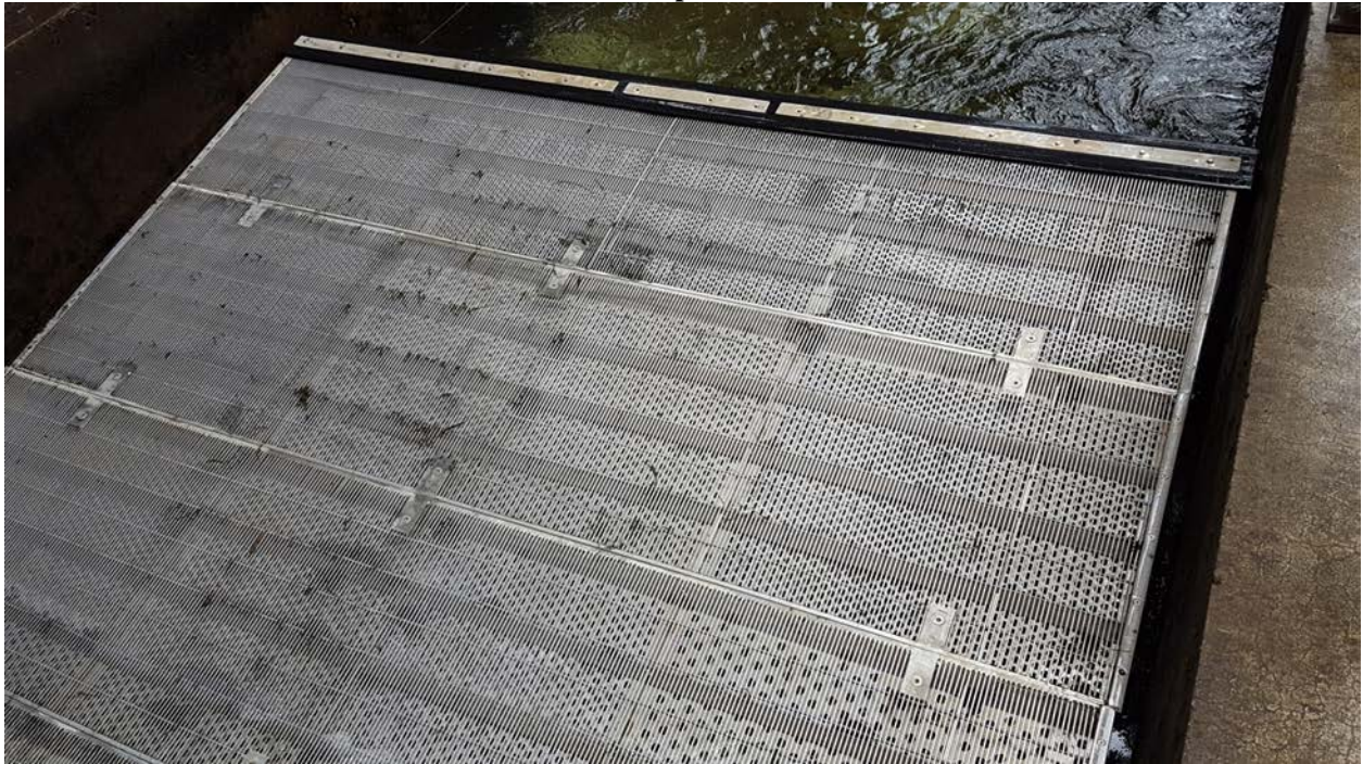
Photo 2. Detail of fish screen and rear-mounted baffle plates
