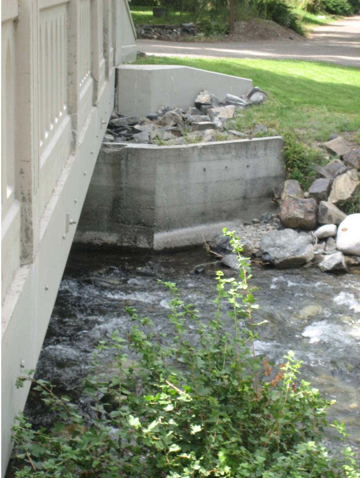
Photo 7: Bailey Lane Bridge, west abutment, downstream face
