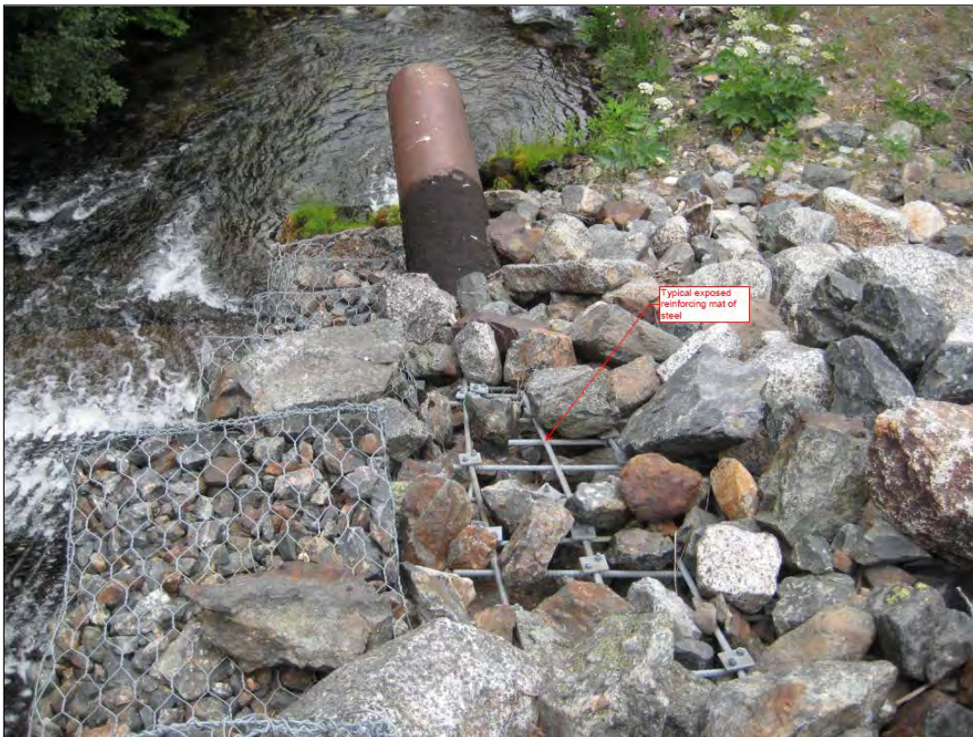
Figure 5. Exposed rebar on dam where rock has sloughed and needs replacement.
