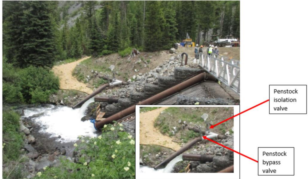
Figure 1: penstock wye with knife gate valves
