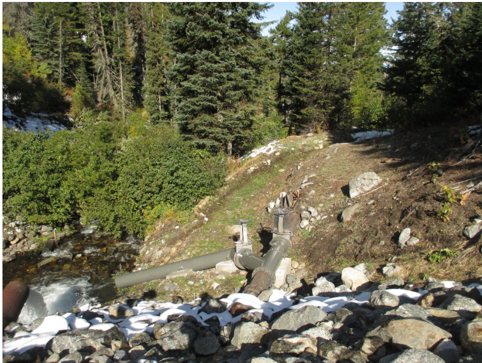
Photo 4 – Penstock wye downstream of Wallowa dam
