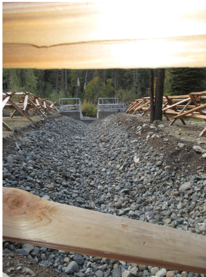
Photo 14 – Tailrace and velocity barrier looking downstream
