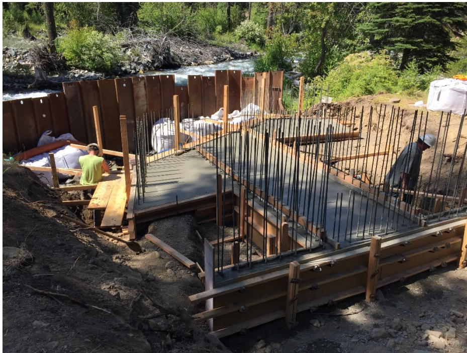
Photo 10 – Fish barrier rebar forms and concrete placement
