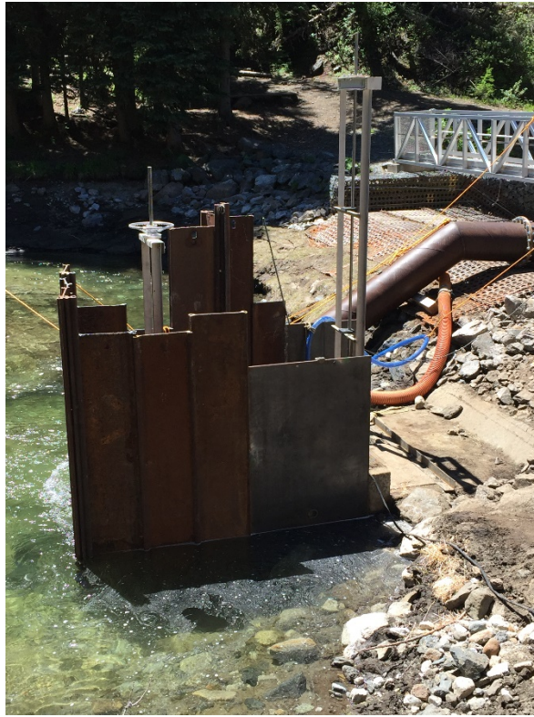
Photo 1 – Cofferdam at Wallowa Falls Intake
