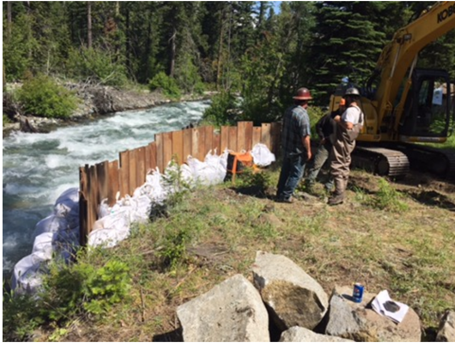
Photo 9 – Cofferdam at tailrace outfall/fish barrier location
