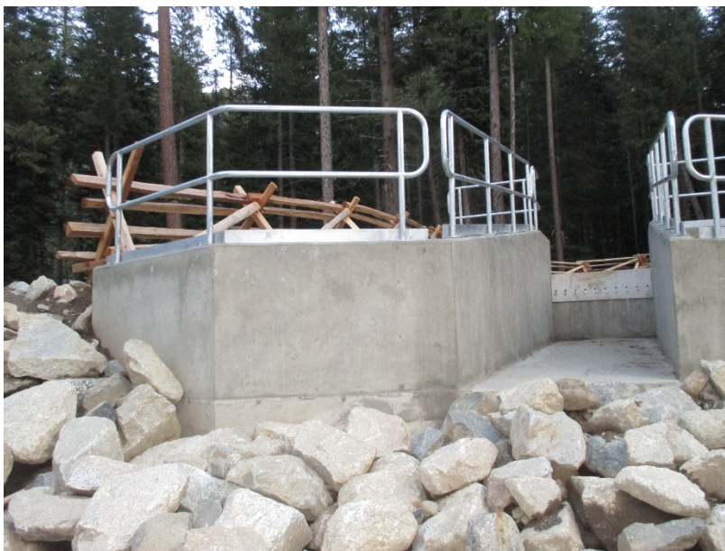
Photo 15 – Velocity barrier looking upstream
