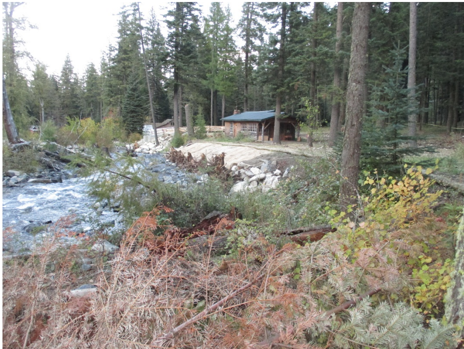
Photo 12 – Completed revetment with revegetation on the West Fork Wallowa River
