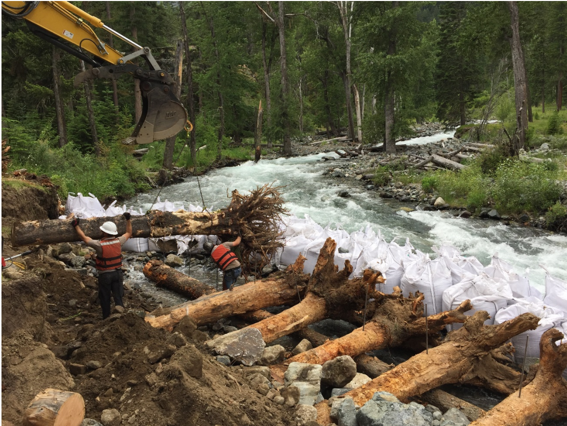
Photo 11 – Cofferdam and log revetment installation
