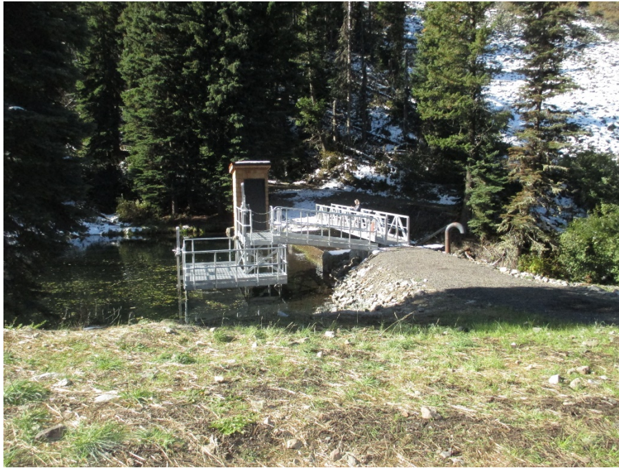
Photo 3 – Completed intake structure and bollards on dam catwalk
