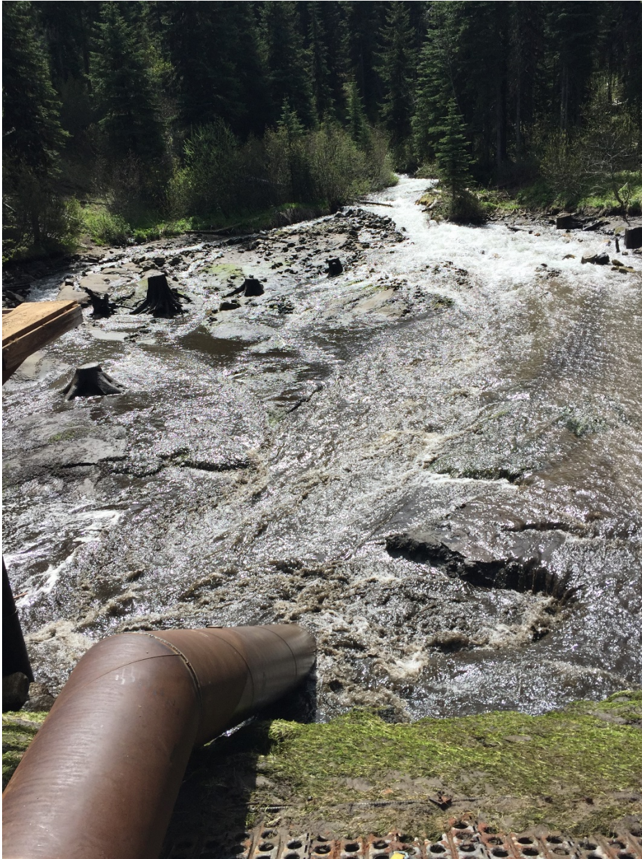
Photo 3 – 20-inch siphon in Wallowa Falls Forebay
