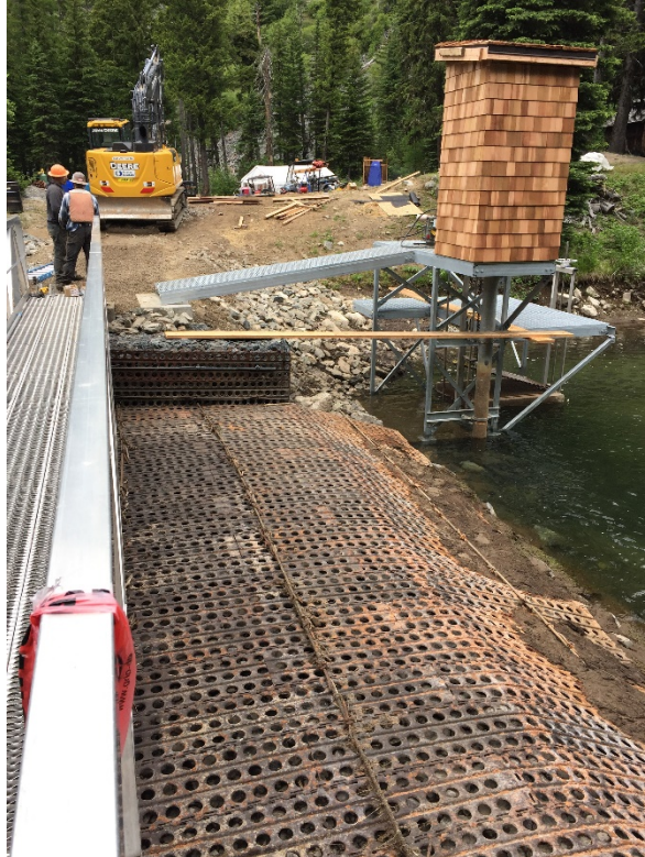
Photo 2 – New Intake Platform
