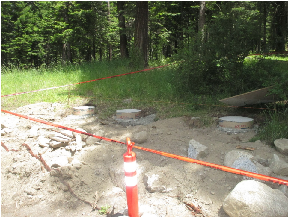
Photo 5 - Foundations for new Eagle Cap Wilderness trailhead sign.
