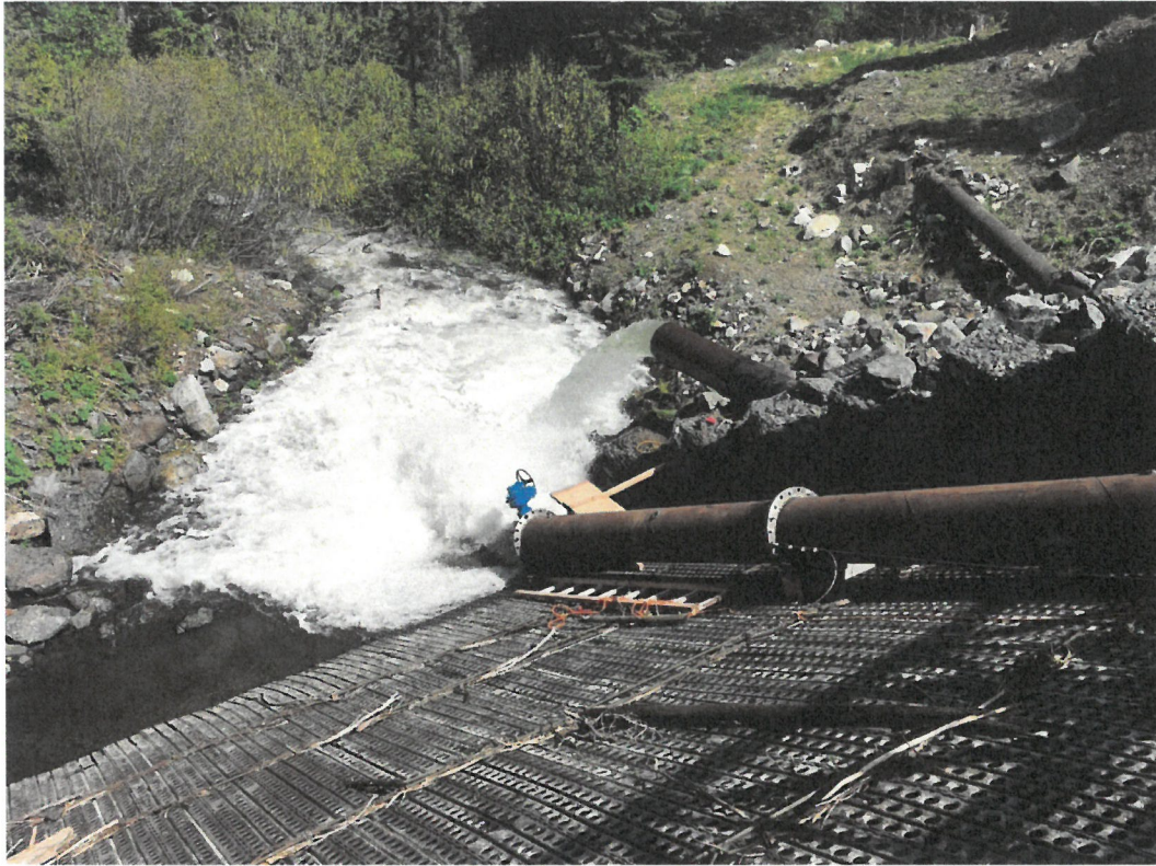
Photo 1 – Wallowa Falls Dam: low level outlet pipe and 20-inch siphon pipe
