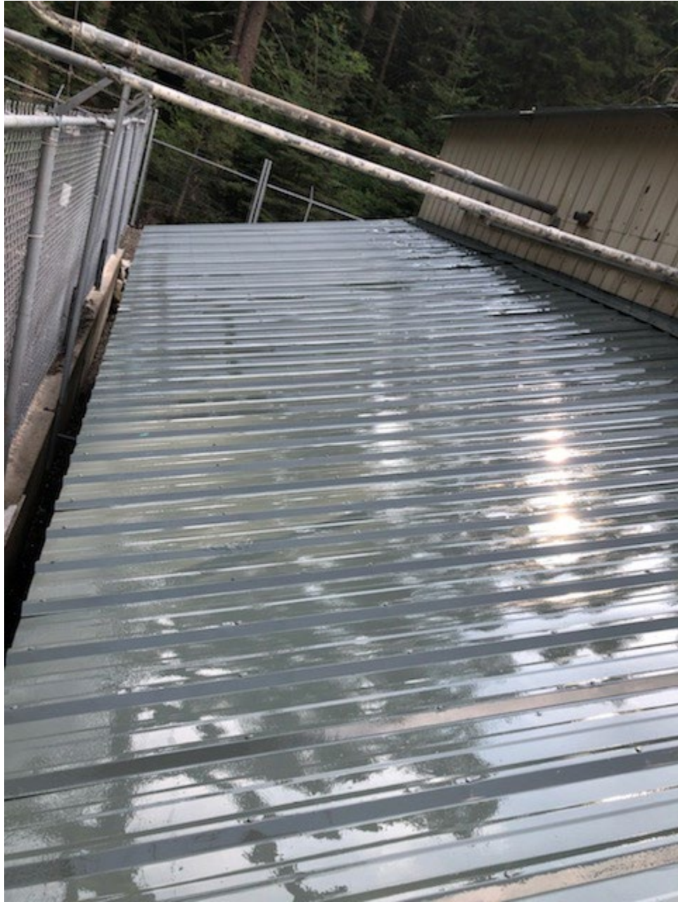
Figure 2: Recoded Powerhouse Roof
