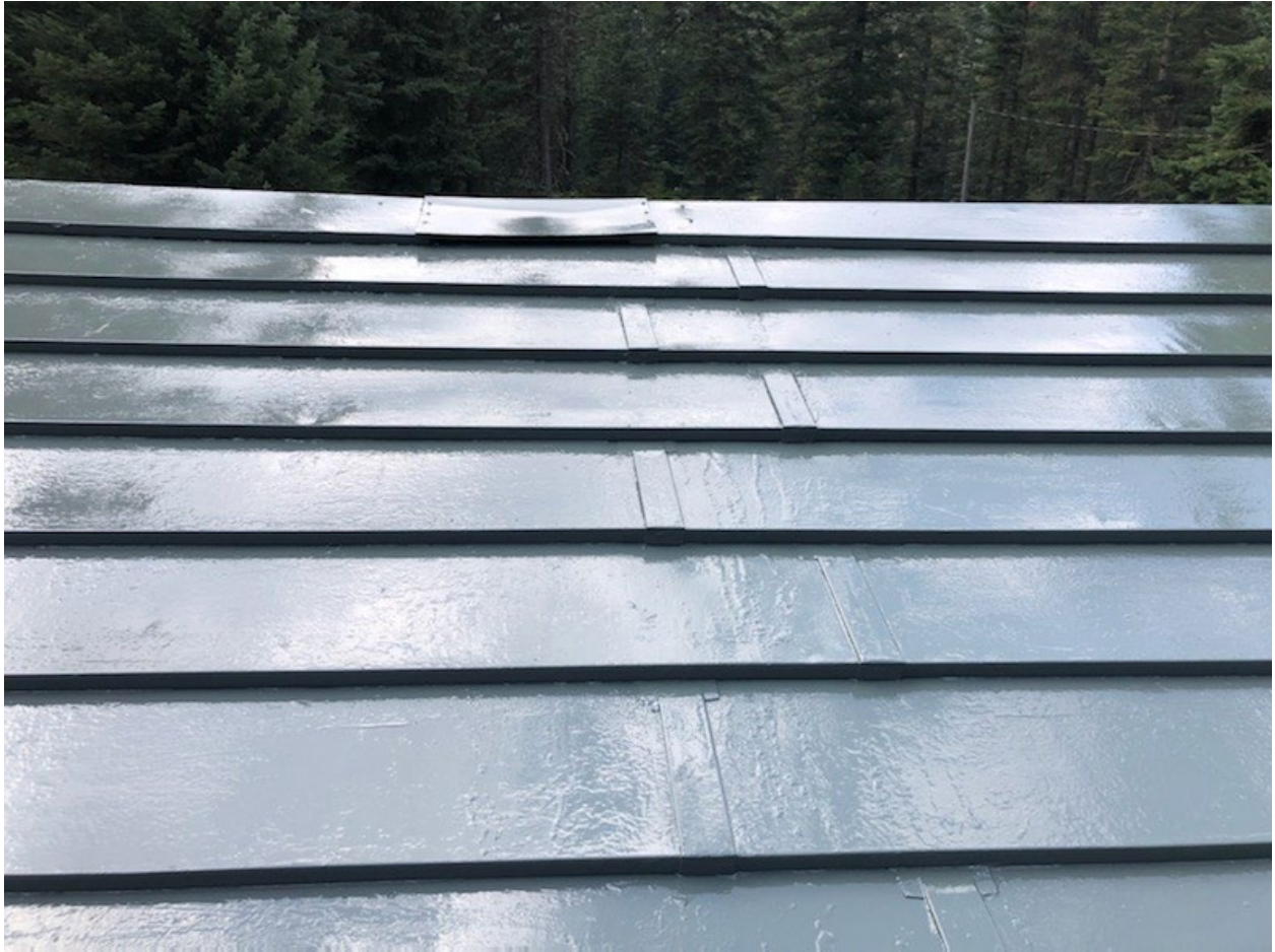
Figure 1: Recoated Powerhouse Roof
