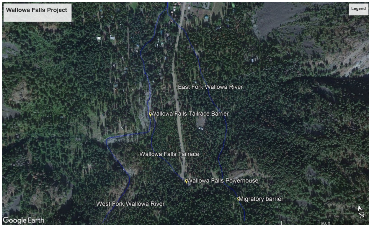
Figure 1 Wallowa Falls Hydroelectric Project.
