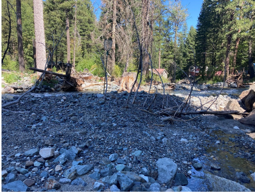
Figure 3. Bottom end of side-channel showing deposited gravel bar and no hydraulic connectivity.
