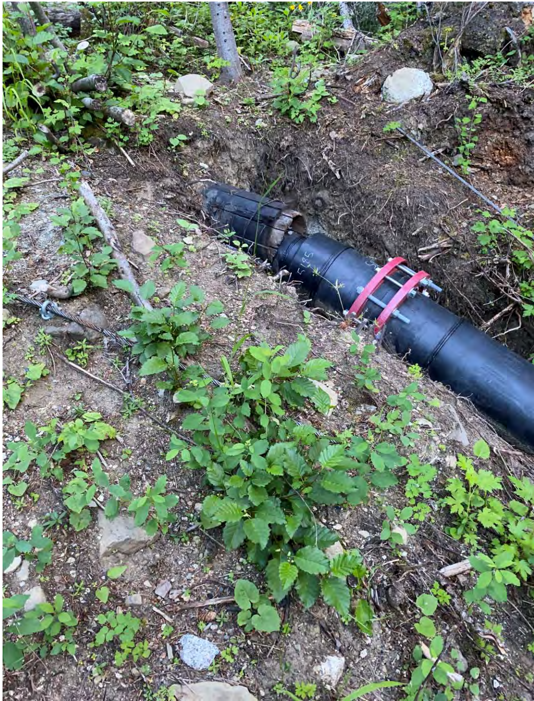
Figure 4. Junction of the existing and new discharge pipe from Royal Purple Creek. (photo- July 27, 2020).
