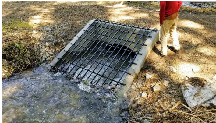
Photo 4: Trash rack upstream of road culvert on lower north tailrace channel (June 5, 2020)
