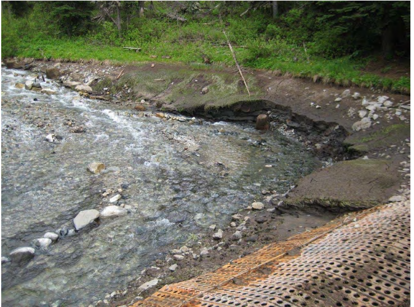
Photo 3 –Wallowa Falls Forebay – some sediment cutting along edges during draining on June 15, 2020
