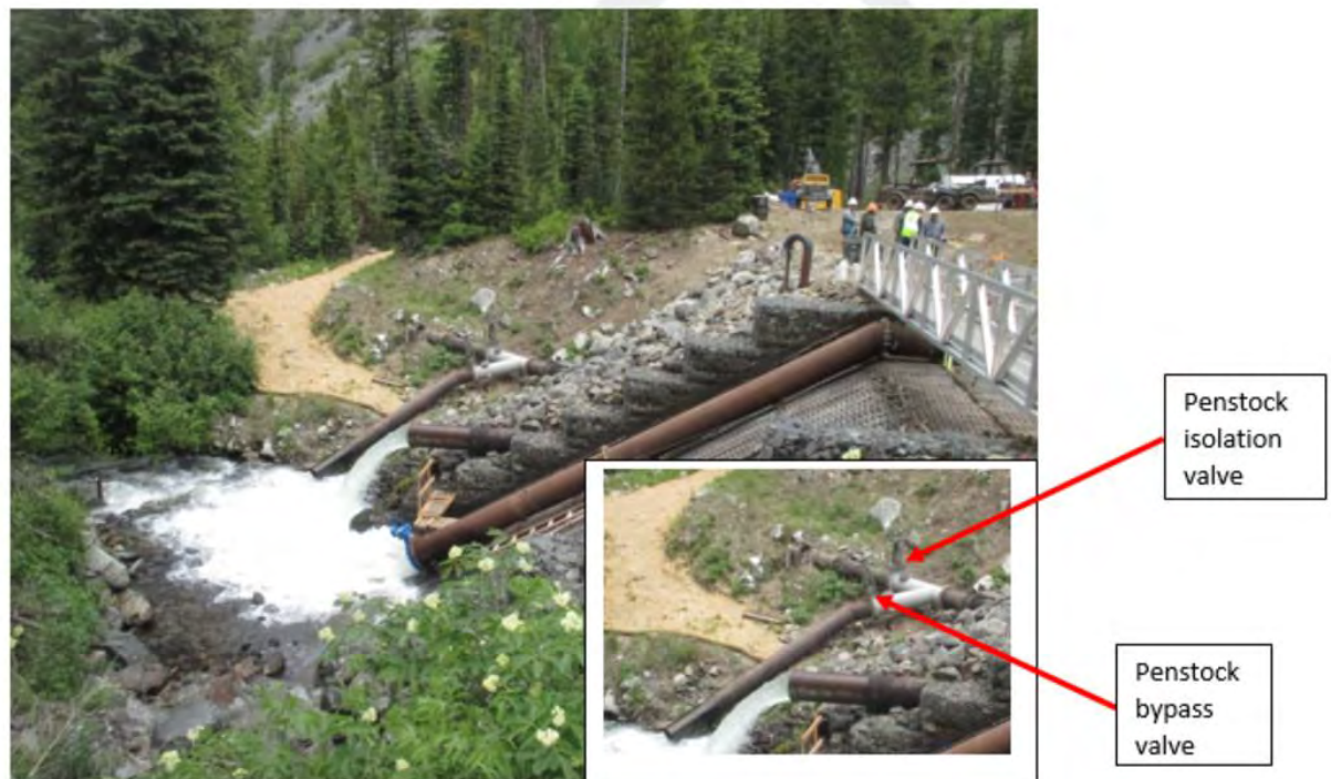
Figure 1: penstock wye with knife gate valves
