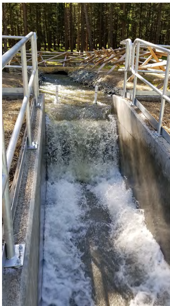
Photo 3: Weir and box flume at tailrace outlet (June 5, 2020)
