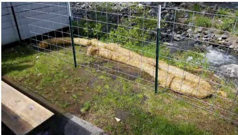
Photo 2: Active discharge and waddle placement to slow runoff into river
