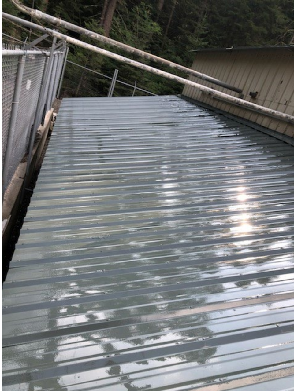
Figure 2: Recoated Powerhouse Roof
