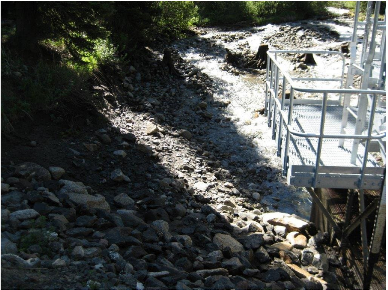
Photo 3:Wallowa Falls Forebay - June 12, 2021
