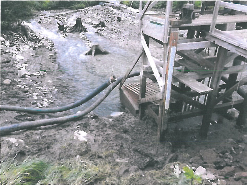
Photo 5 – Channels dredged out to increase sediment transport out of forebay
