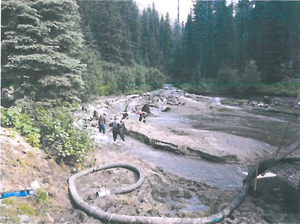
Photo 3 – Crew working to direct stream flow for sediment transport
