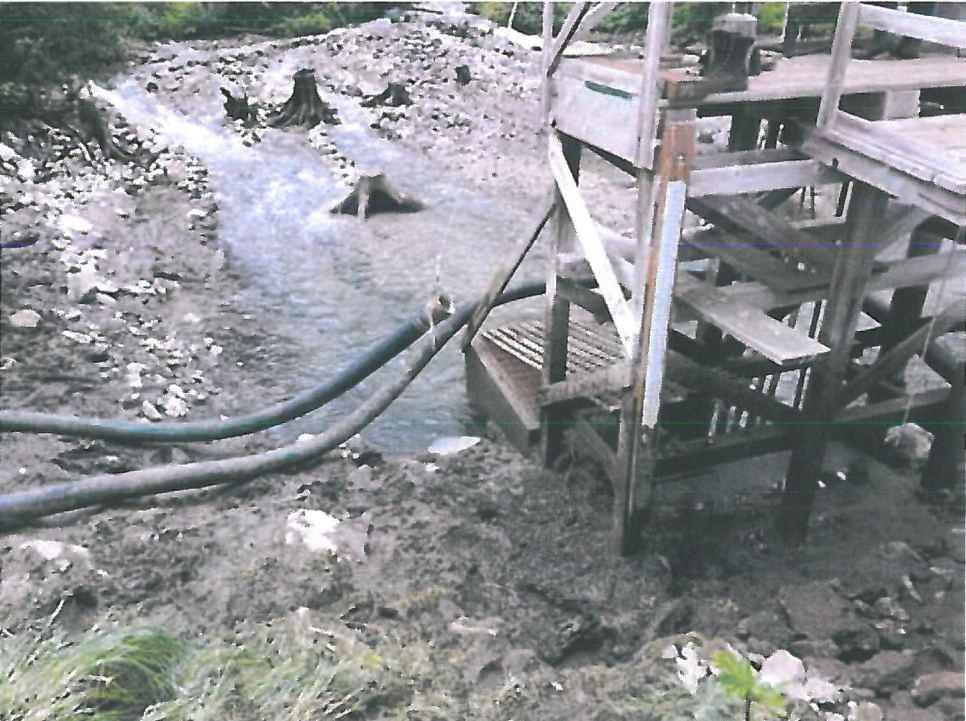
Photo 6 –Forebay after dredging and flushing operation
