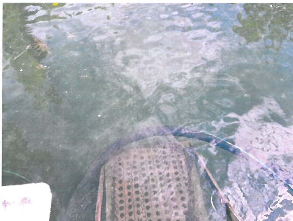
Photo 2 – Dredge hose upstream of penstock intake
