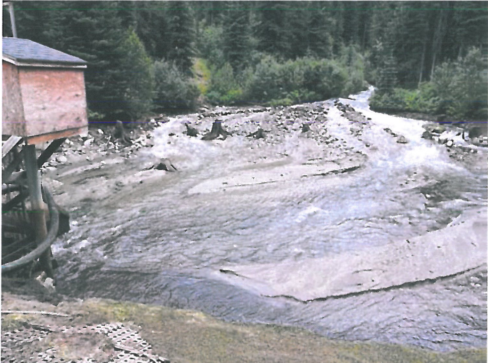
Photo 4 – Stream flow through forebay redirected using rocks in forebay
