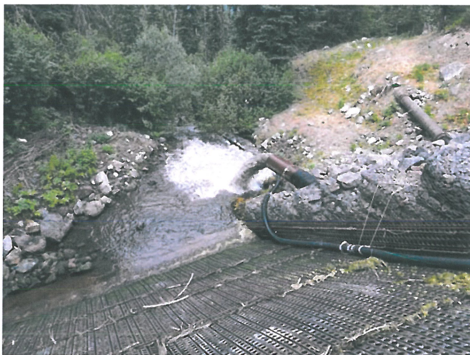
Photo 1 – Dredge hose installed over spillway
