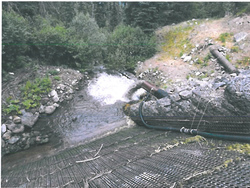
Photo 1 – Dredge hose installed over spillway
