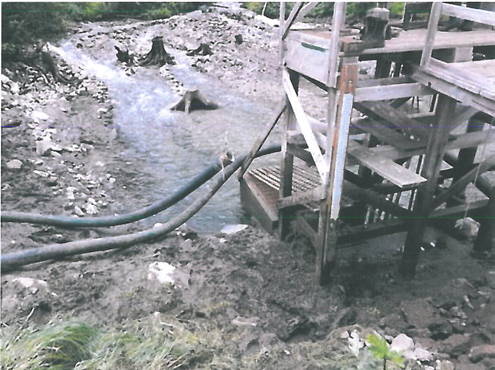
Photo 6 –Forebay after dredging and flushing operation
