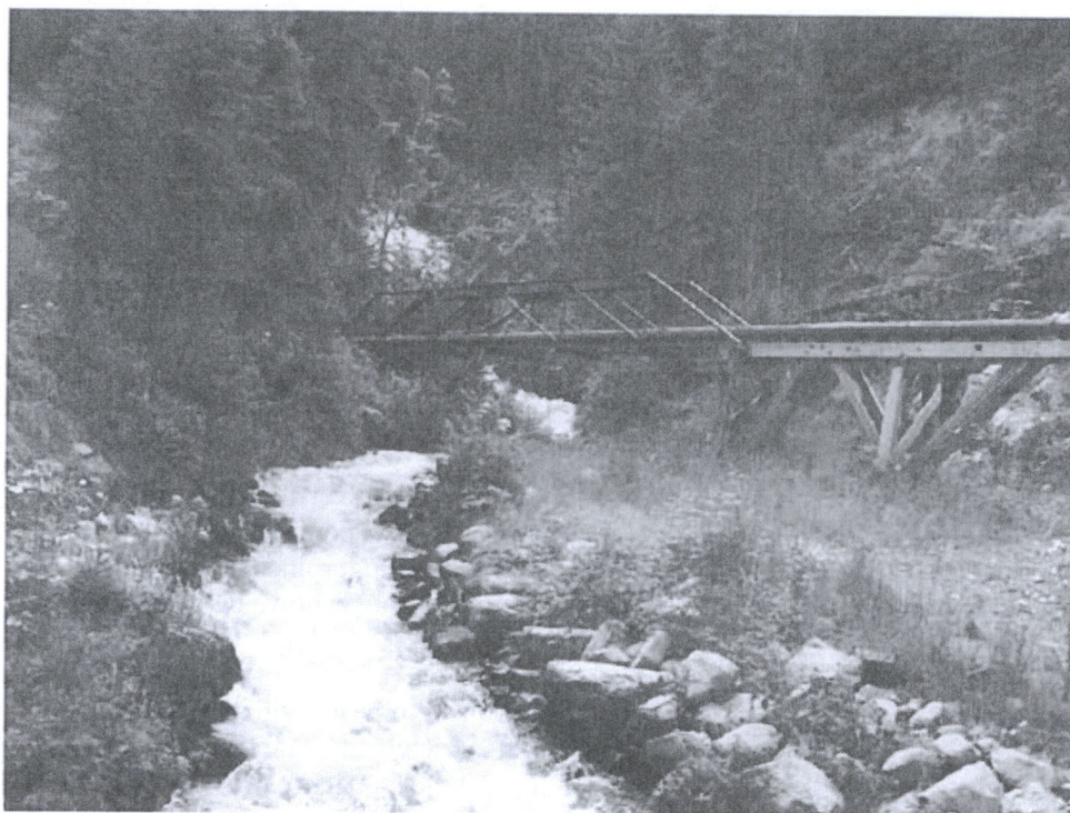
Figure 10: Project penstock crossing over by-passed reach of East Fork Wallowa River. (PacifiCorp, 2011)
