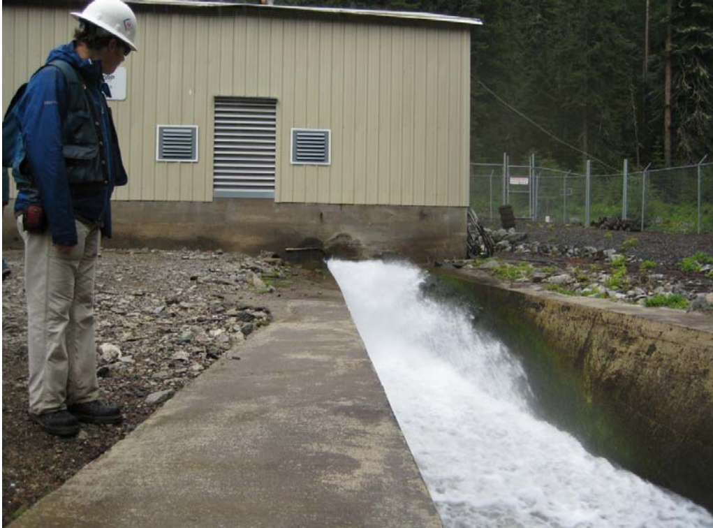
Photo 25: Project Powerhouse and Tailrace
