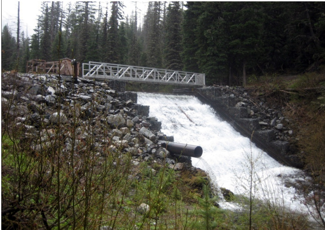
Photo 5: Project Dam, Spillway and Catwalk
