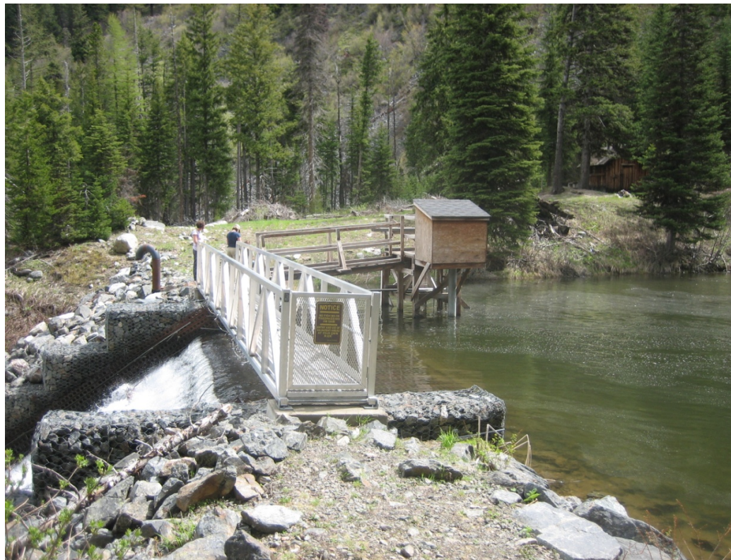
Photo 6: Project Spillway, Dam, Catwalk, and Intake Structure
