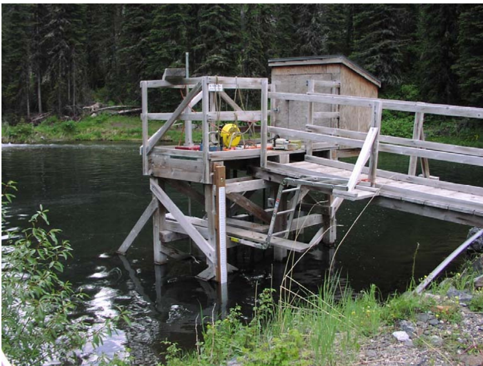
Photo 4: Project Forebay and Intake Structure
