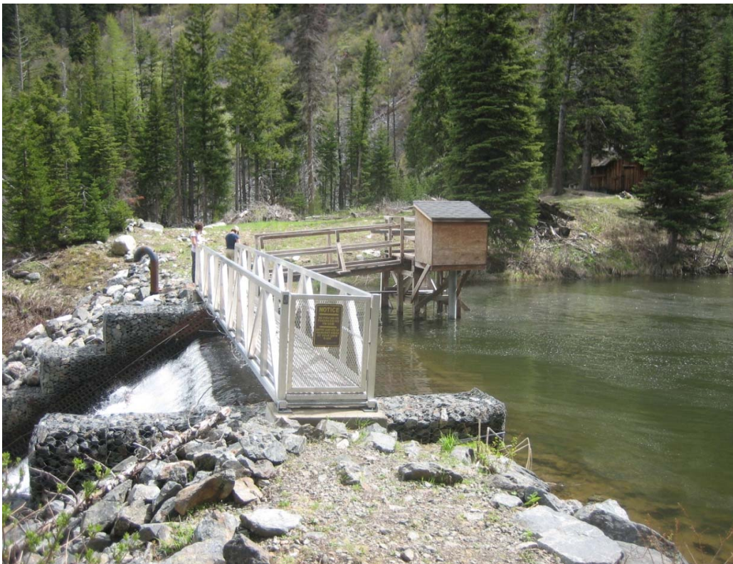
Photo 6: Project Spillway, Dam, Catwalk, and Intake Structure
