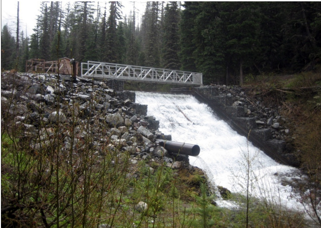
Photo 5: Project Dam, Spillway and Catwalk
