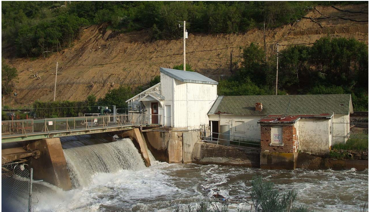
Photo 2. Diversion Dam and Intake Street Level View
