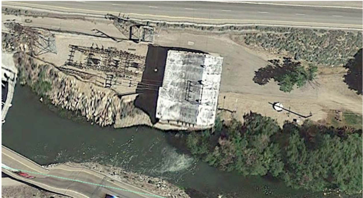
Photo 4. Aerial View of Powerhouse and Substation (Substation is not part of the Project)
