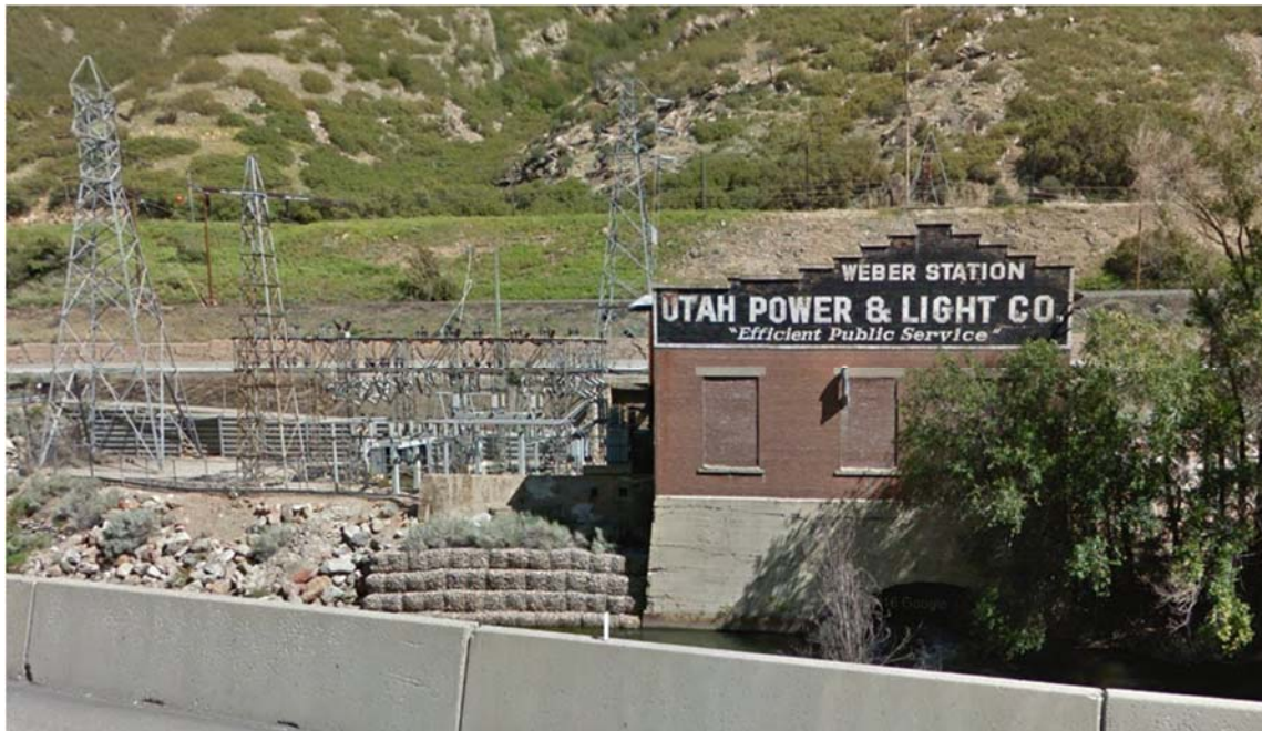
Photo 5. Street Level View of Weber Substation (Not part of the Project) and Powerhouse
