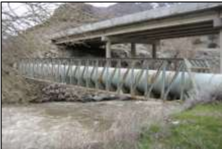
Figure 11. Pipeline trestle river crossing with I-84 in the background.
