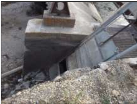
Figure 6. Fish ladder with slide gate opening, calibrated annually for minimum stream flow.
