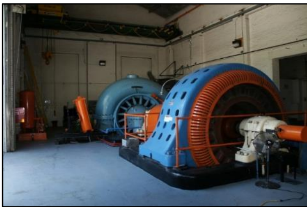
Figure 19. Generating unit in powerhouse.
