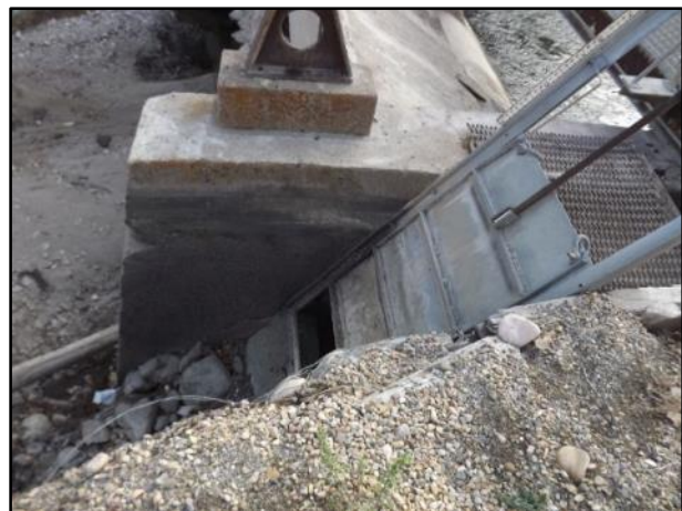
Figure 6. Fish ladder with slide gate opening, calibrated annually for minimum stream flow.
