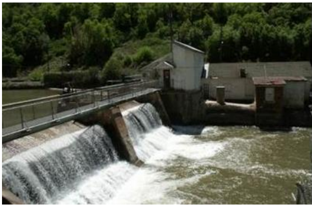
Figure 7. Weber diversion dam spilling; intake house and beginning of flowline visible.
