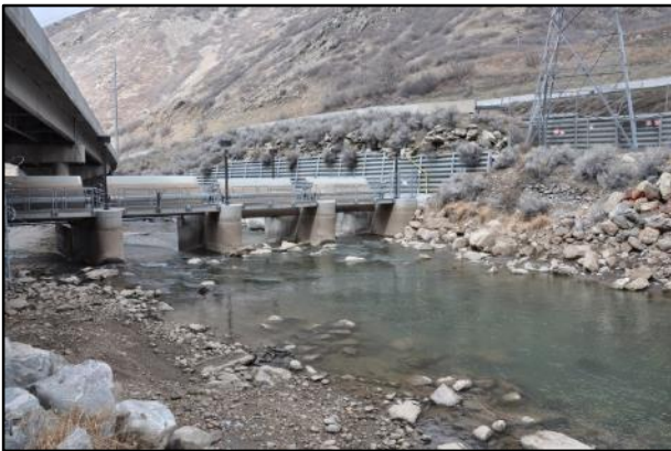
Figure 21. Weber-Davis Irrigation Company diversion dam under I-84; gates open.
