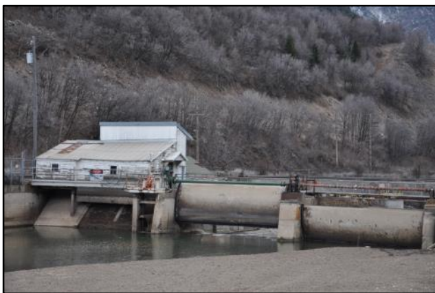
Figure 9. Weber project diversion dam radial gates; forebay de-watered.
