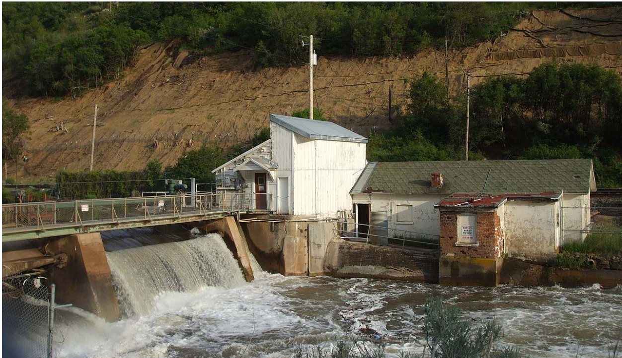
Photo 2. Diversion Dam and Intake Street Level View
