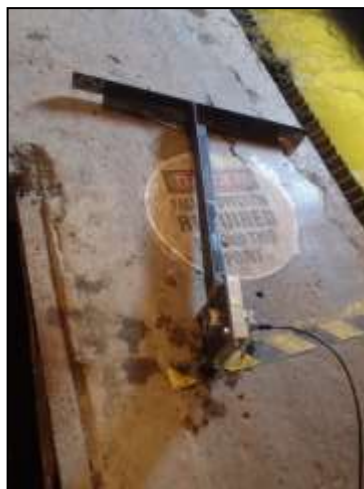
Photograph 2. Relocation of the camera between intake rack and penstock gates.
