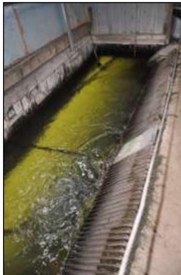
Photograph 7. Project intake trash rack. Bar spacing is 1.25 to 1.5 inches.
