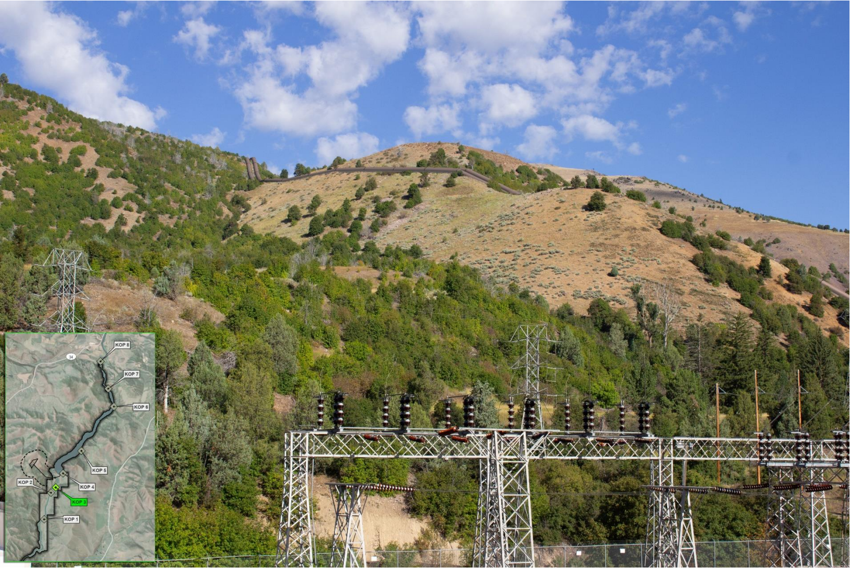
KOP 3 – From Oneida Road looking across Oneida Substation
