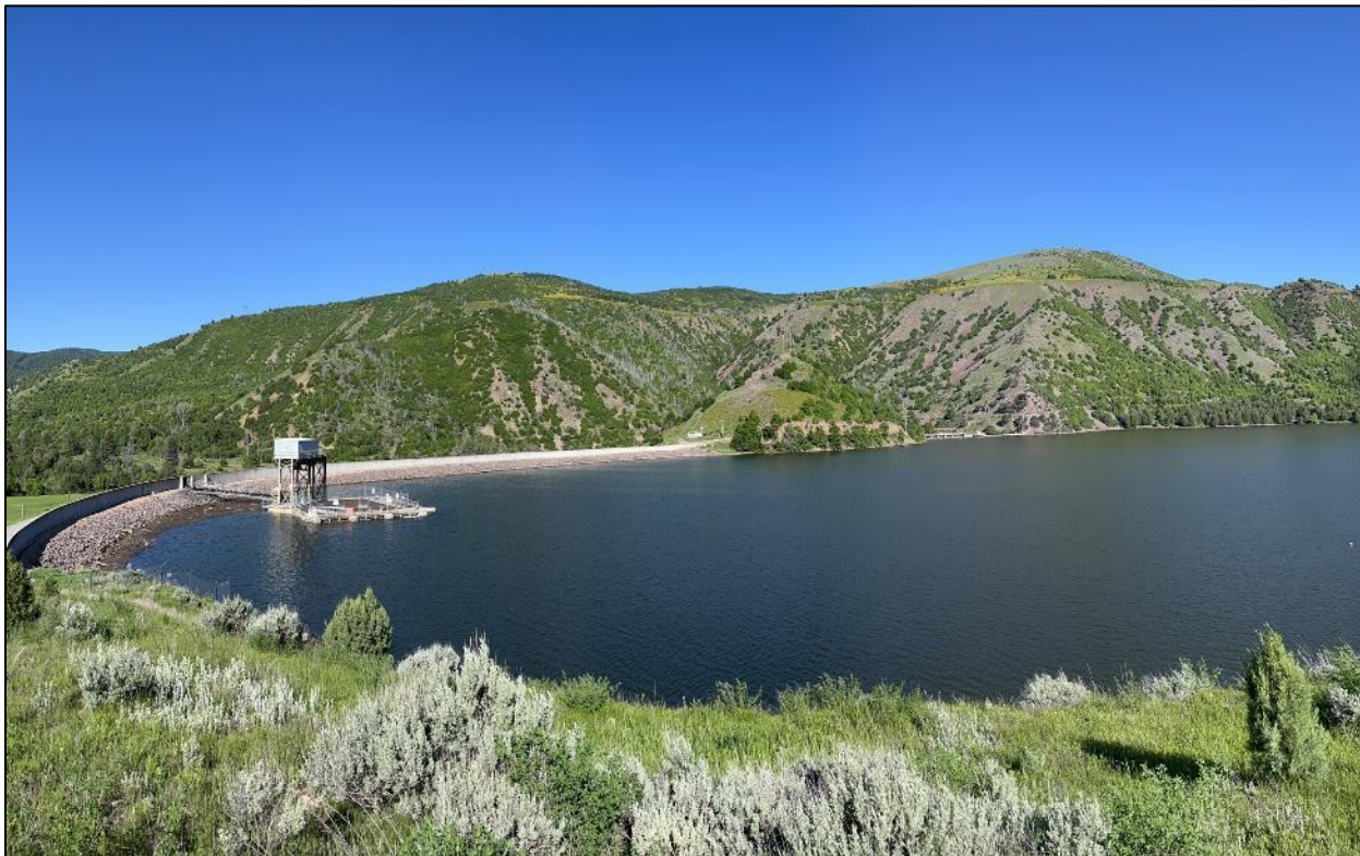
Figure 4.2-7. Oneida Reservoir shoreline with bank armoring around the embankment dam.
