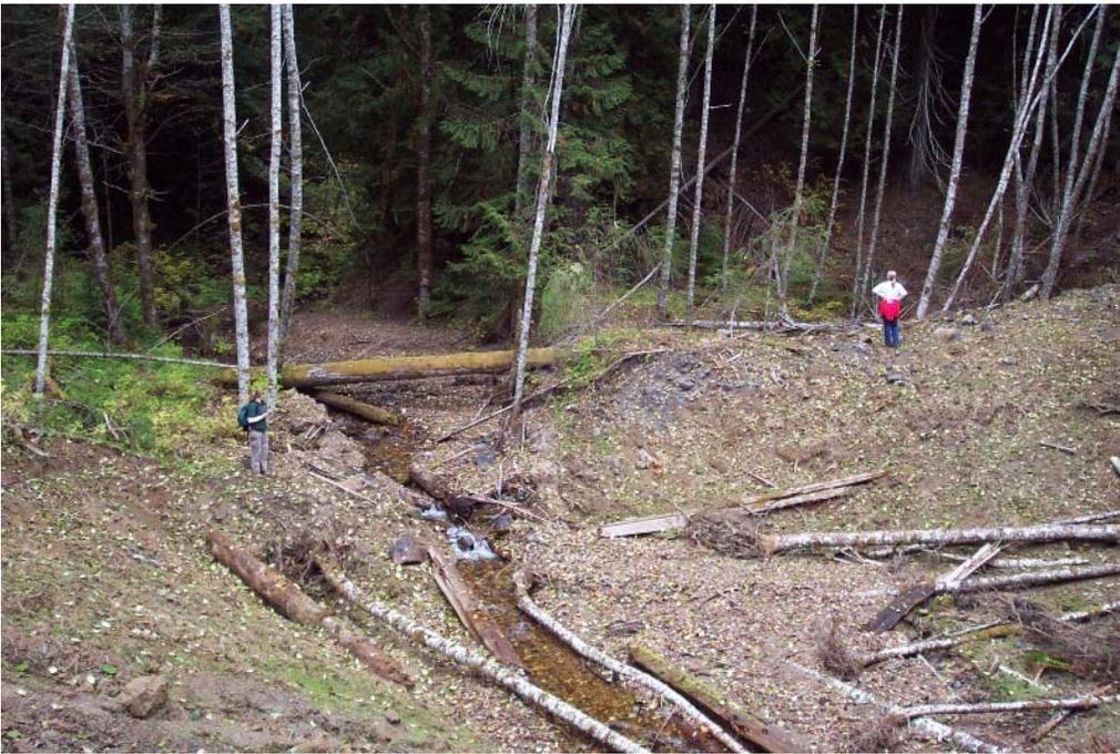
Figure 5. Fish Bearing Stream "A" after culvert removal and reshaping streambanks
