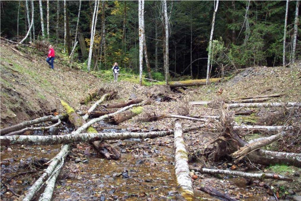
Figure 6. Fish Bearing Stream "B" after culvert removal and reshaping streambanks
