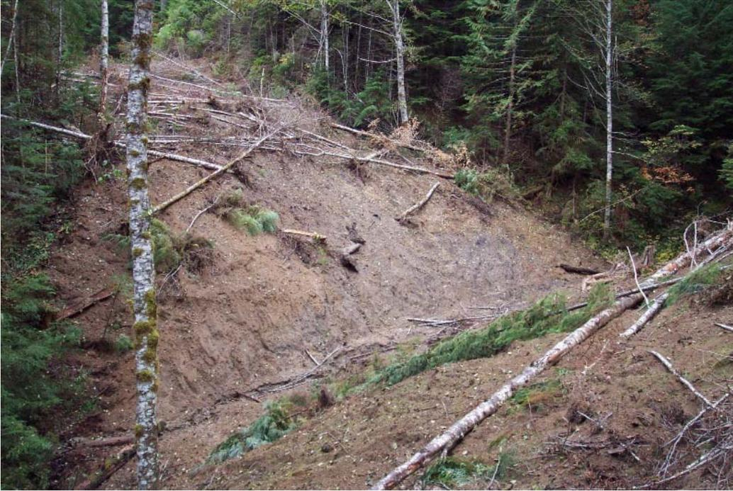
Figure 8. Culvert Removed from intermittent stream and streambanks reshaped
