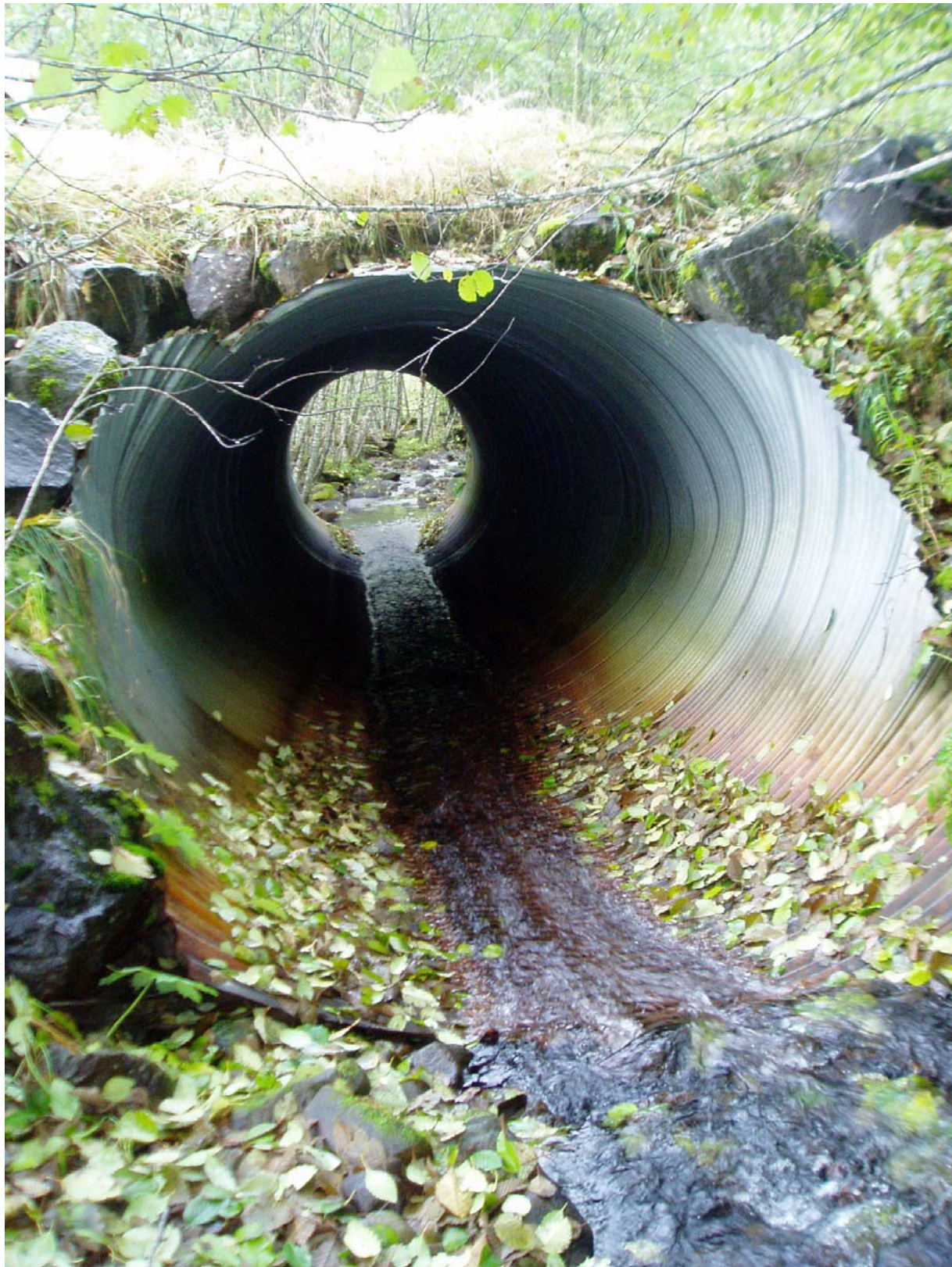
Picture 2. Inlet of culvert to be replaced. Tracy 2005
