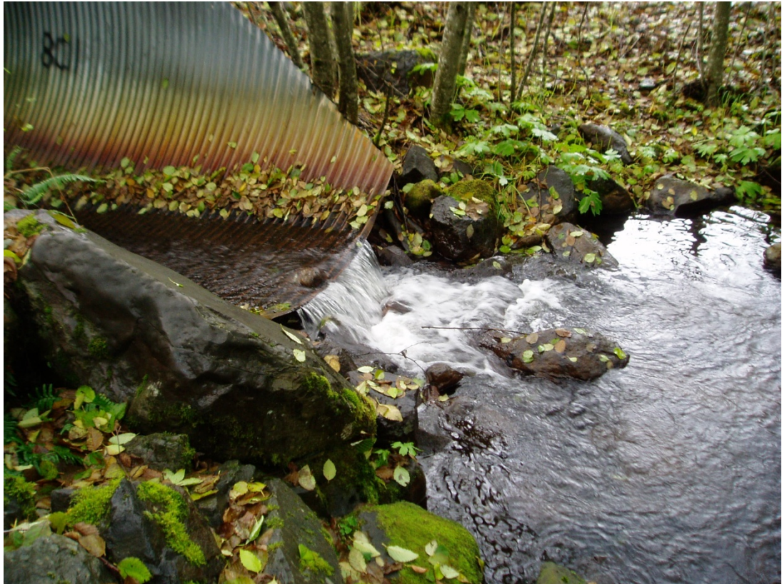
Picture 1. Outlet of Culvert to be replaced. Tracy 2005
