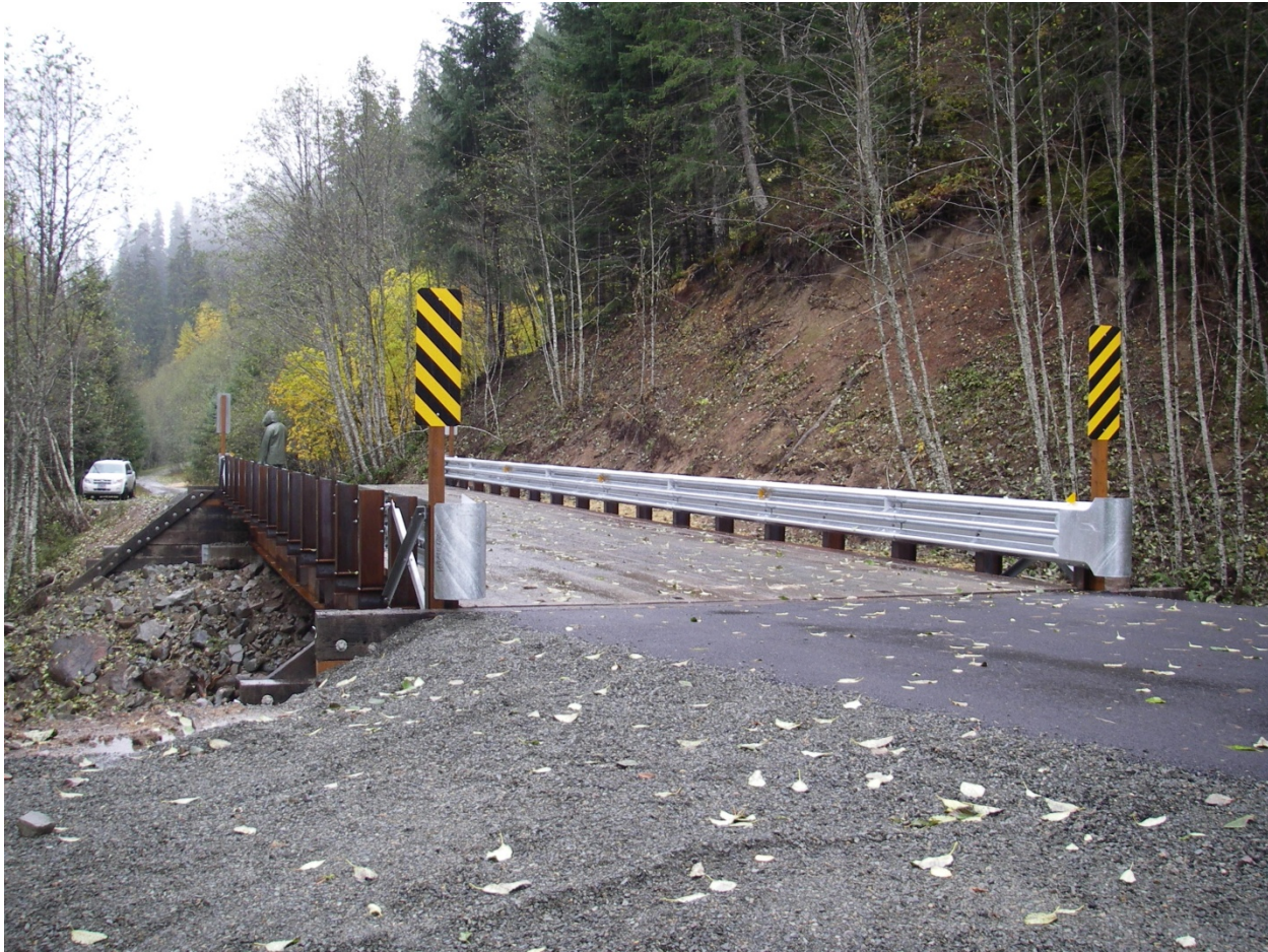
Picture 4. New bridge in place of old culvert. Becker 10/2009
