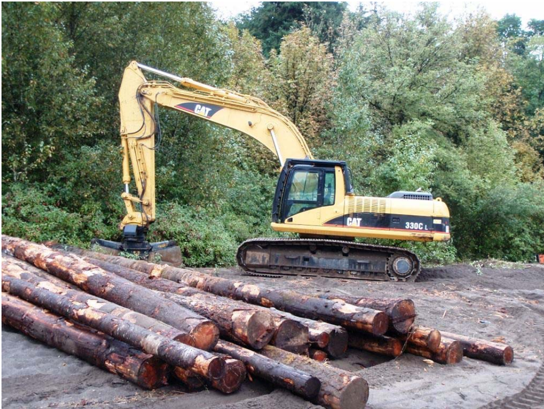
Pilings being staged (Photo: Shannon Wills)
