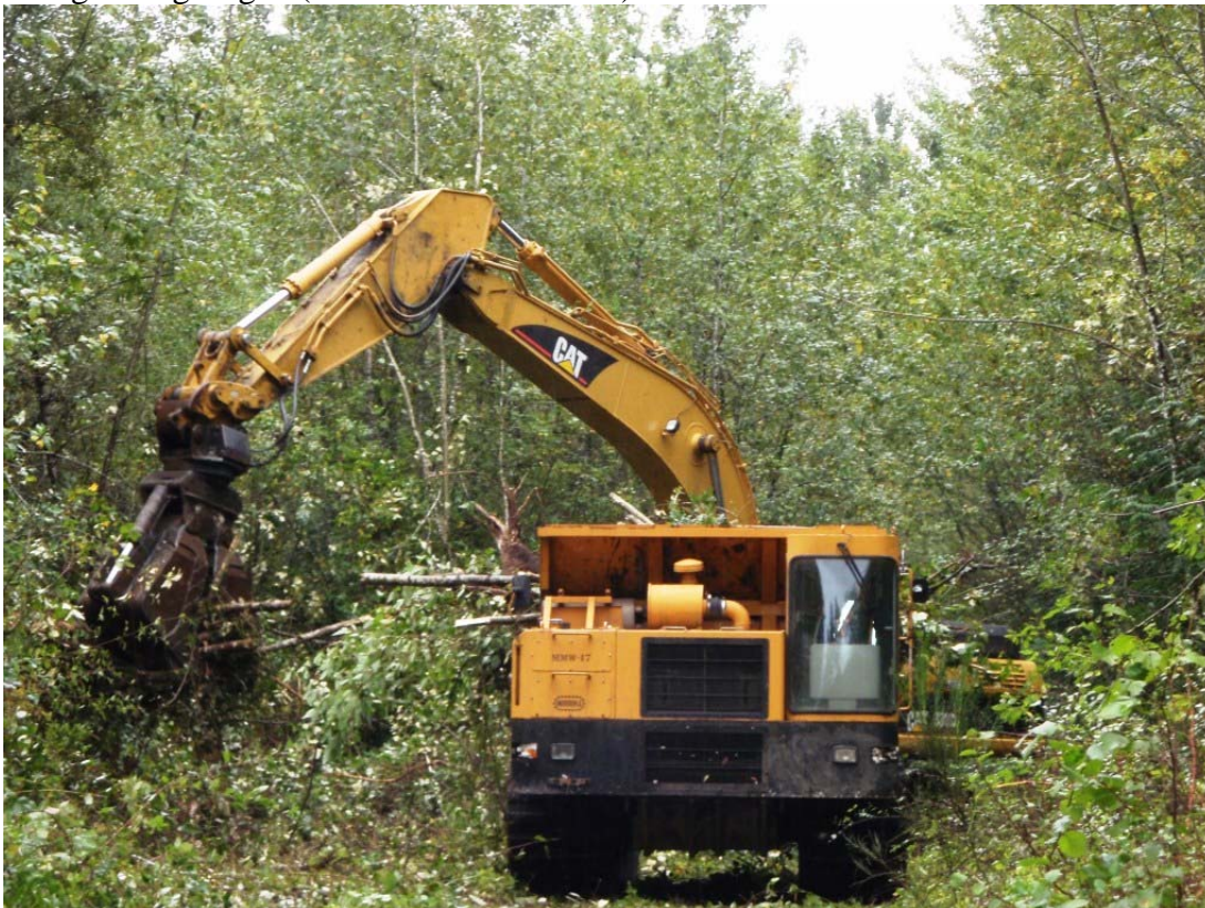
Brush and debris being collected on-site for use in the ELJ (Photo: Shannon Wills)
