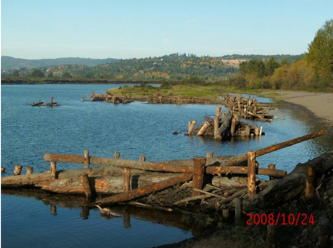
All seven completed ELJ at high tide during the end of the low-water season. (Photo: Tony Meyer [Oct 24 2008])
