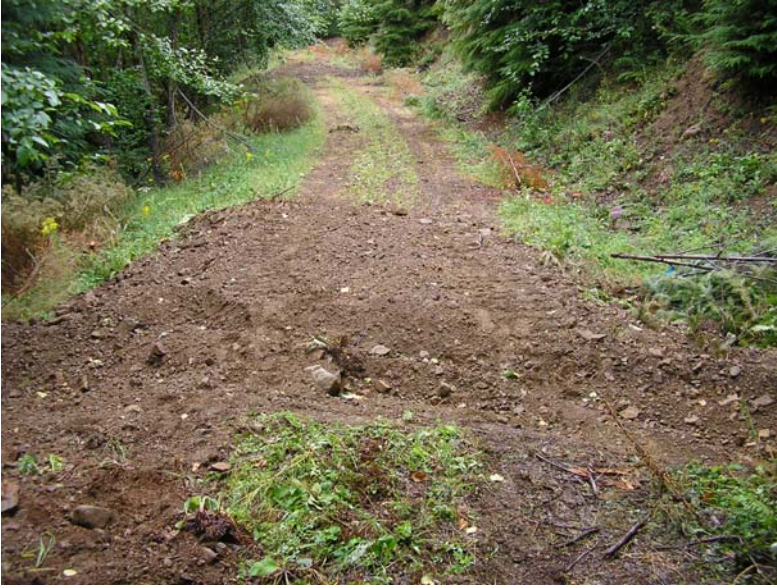
Road Ditching, Kirk Naylor, August 2008
