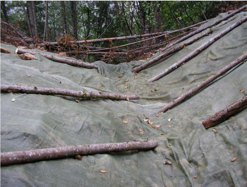
Erosion Control, Kirk Naylor August 2008
