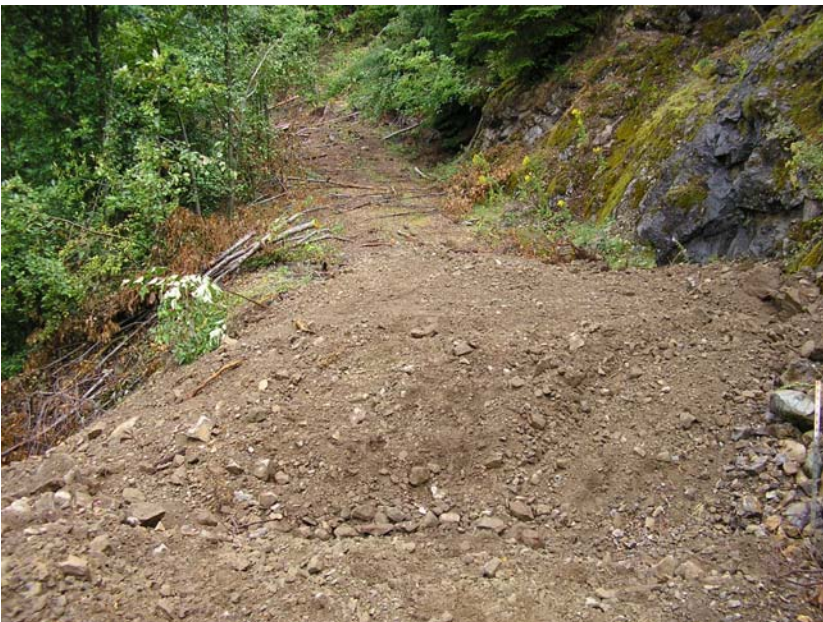
Culvert Removal, Kirk Naylor, August 2008
