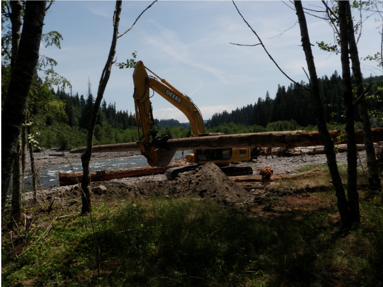
2. Streambank stabilization structure under construction
