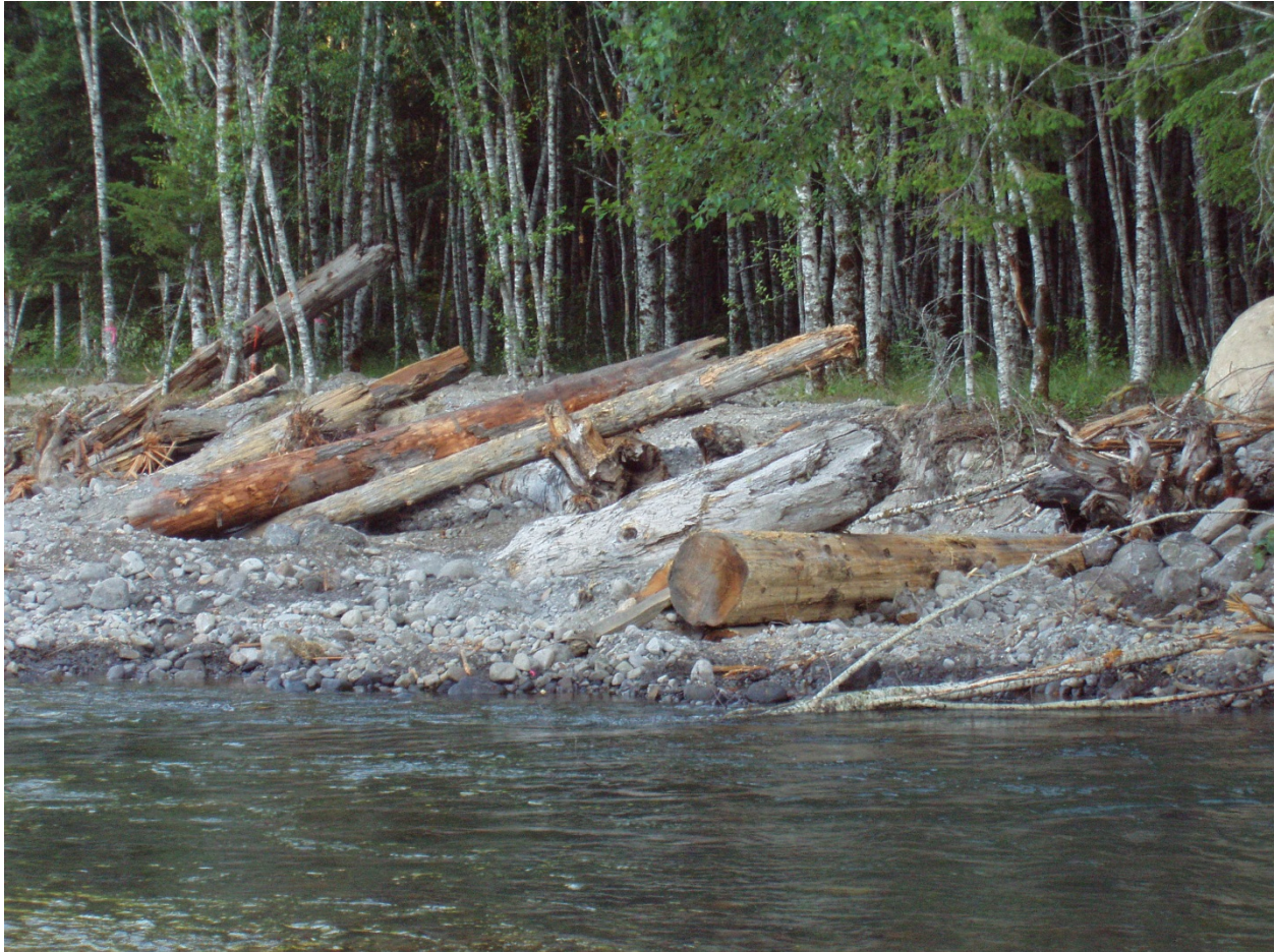
4. Completed streambank structure
