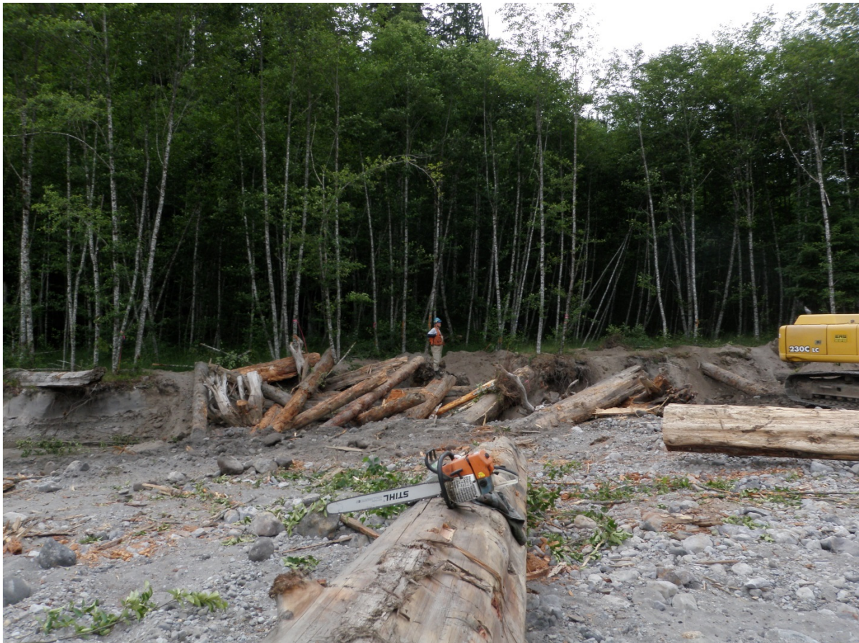
1. Streambank stabilization structure under construction
