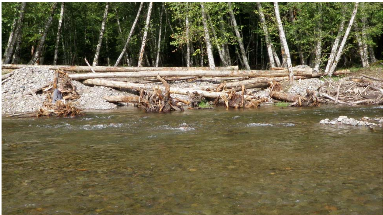
A series of 4 structures with 31 logs were placed at ST#16. Coho were observed spawning and rearing in and around the structure in fall 2011.
