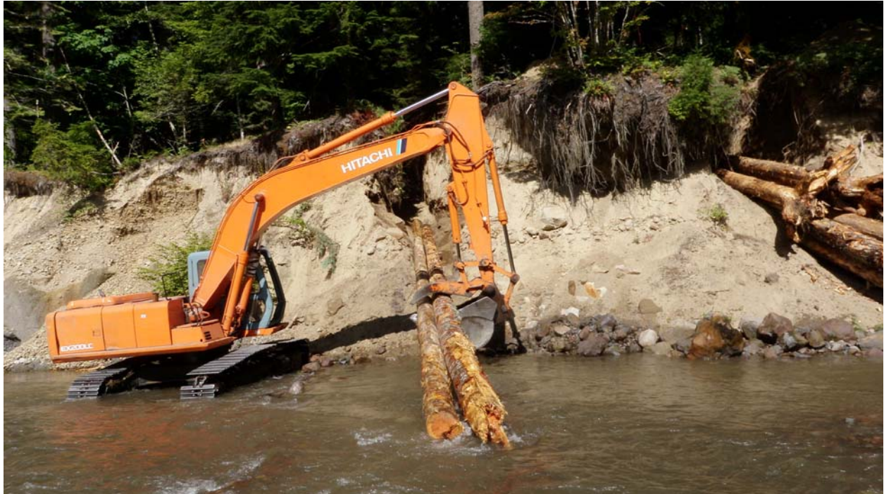
Excavator placing logs into banks ST#10
