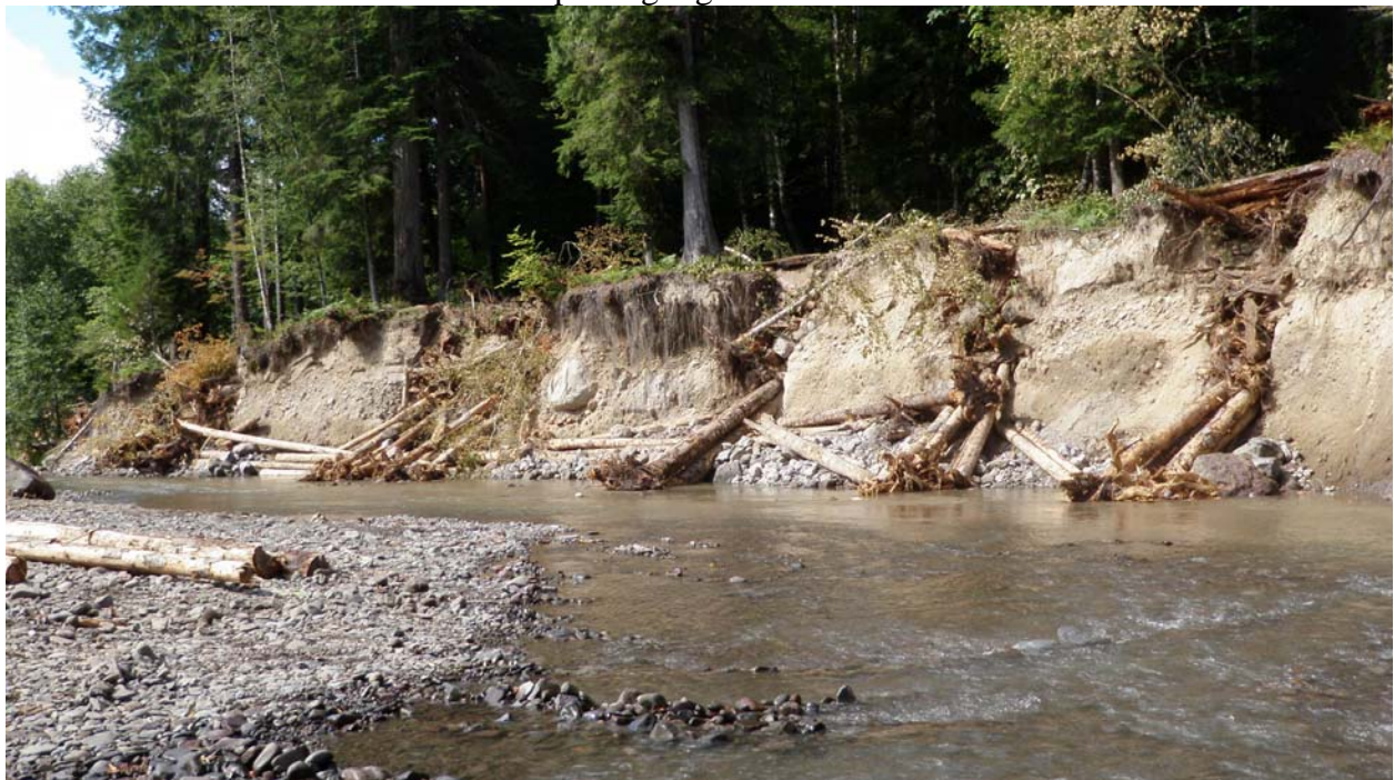
Completion of bank stabilization 87 logs was placed in eroding banks. Gravel bar on river left was shaved back 15-20 feet to help reduce flow on banks. ST#10
