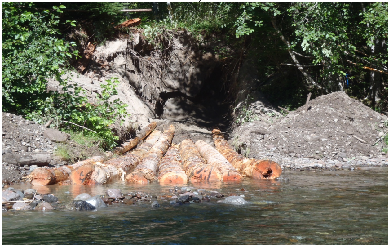
Logs buried 30-40 feet to increase stability, 7 logs in structure so far, a 5ft deep scour pool was created with this structure. Coho have were observed using this structure.
