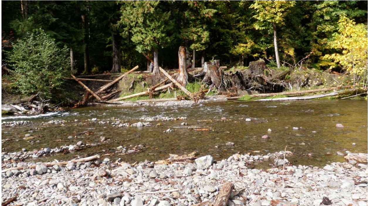
Looking across after construction of bank stabilization project 21 logs in ST#15
