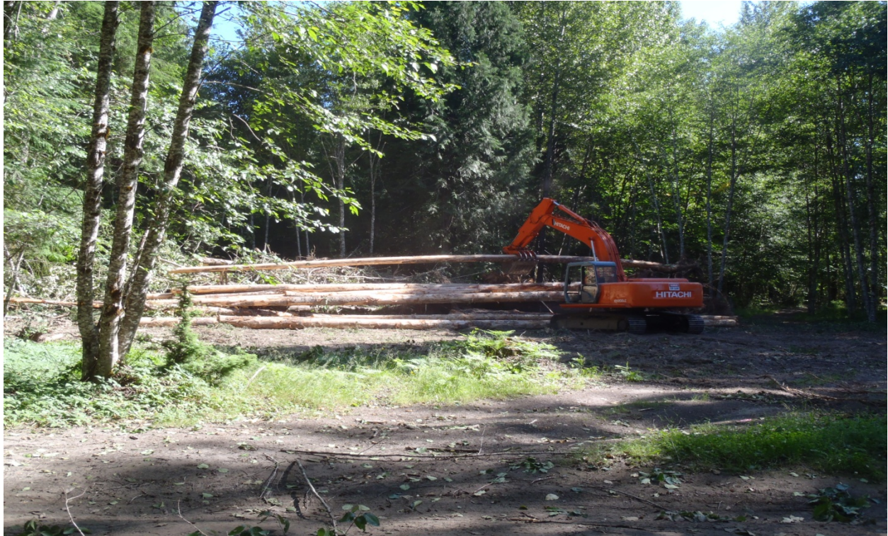
Stockpiling logs at the staging area
