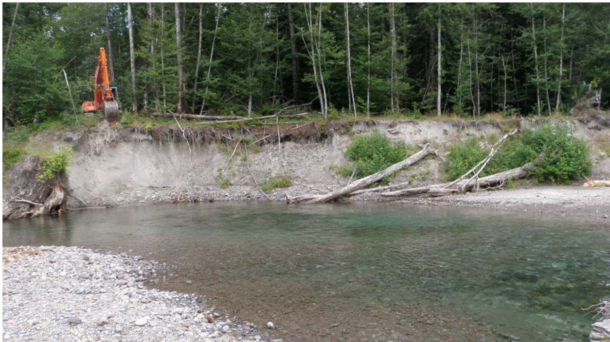
Looking down stream at eroding bank prior to bank stabilization structure ST#2
