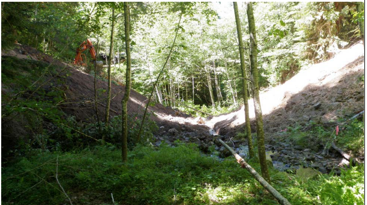
Picture 2. Largest culvert removed 9300150 road. Michaelis 7/20/2010
