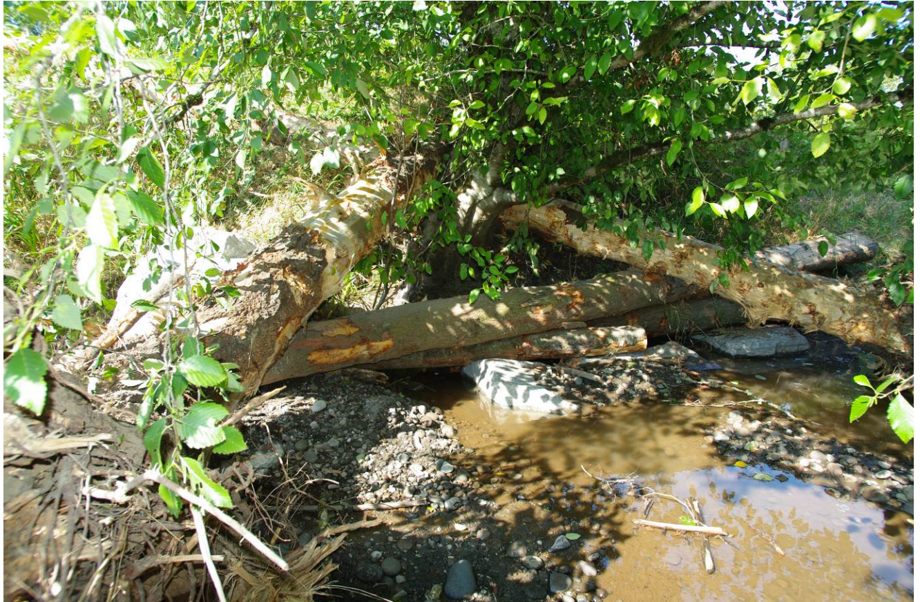
Incorporating an existing alder to make a habitat wood structure
