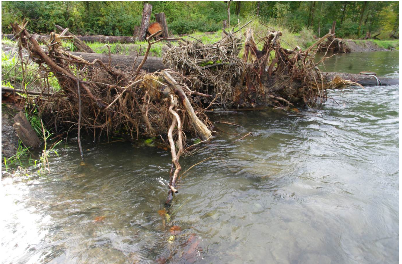
Scour pool structure after
