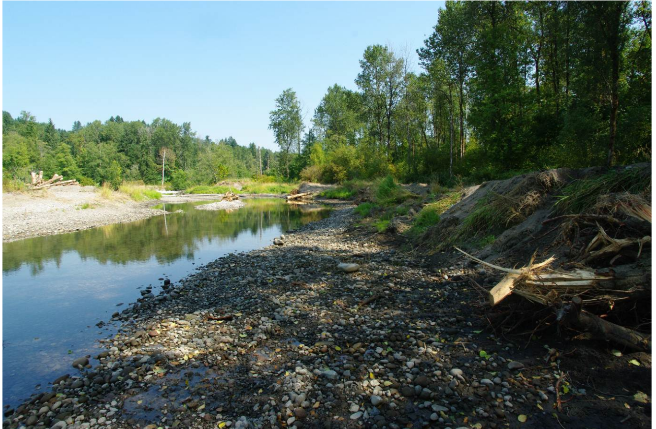
Looking upstream from the south bank of the side channel from the pre-construction photo. Visible on the right are three scour pool structures, in the center a log with rootwad anchored in place, and the head end apex bar jam on the left. Floodplain wood is not yet in place.
