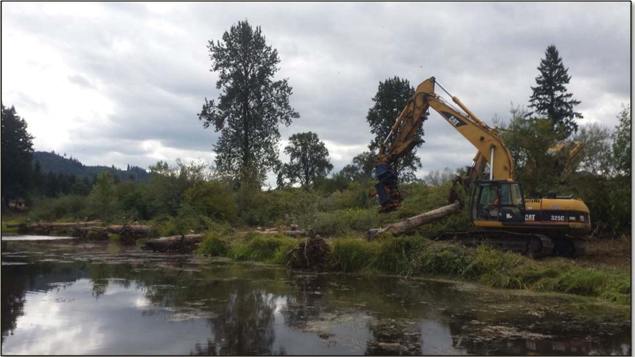
Looking downstream at Site C during construction.
