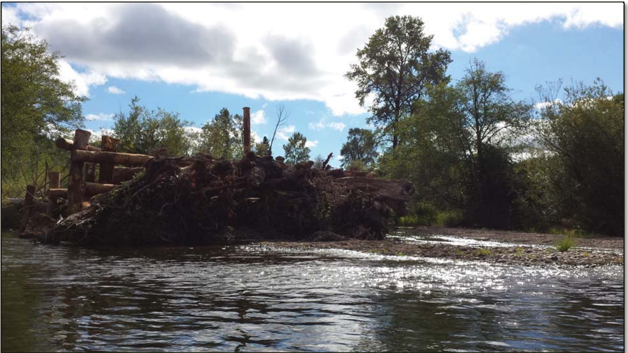
Looking downstream at Site C apex jam with reconnected water flow to the right of the picture.
