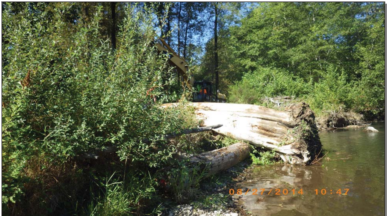
Apex jam location as first wood is placed at Site B.
