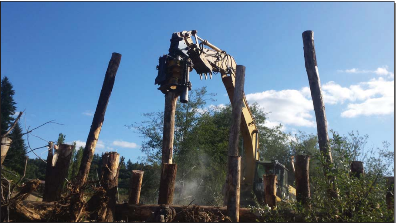
Apex jam during Site C construction.
