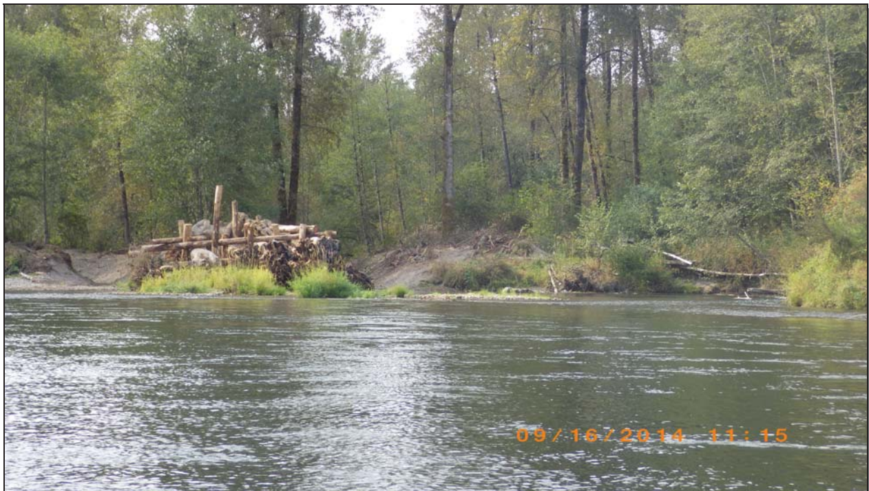
Site B apex jam with side channel entries excavated to the right and left of the structure.
